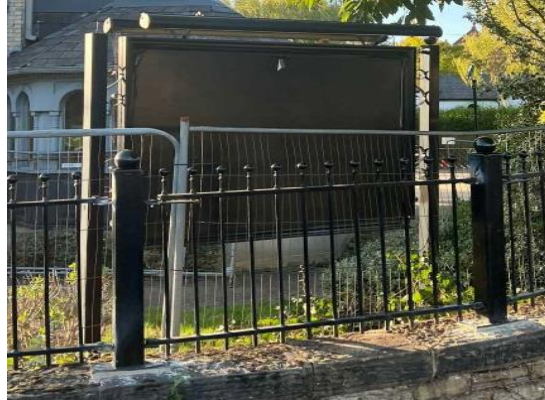
Figure 6: Existing advertising board to the front corner of the site
