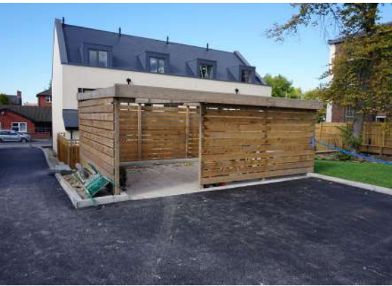
As built timber refuse store on site.
