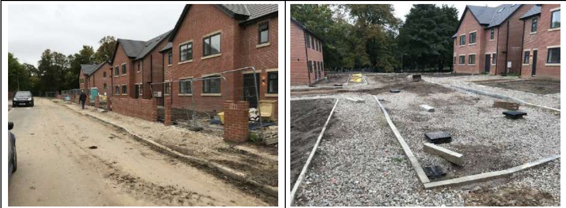
Photographs 1-2: Site photographs showing site almost complete.
