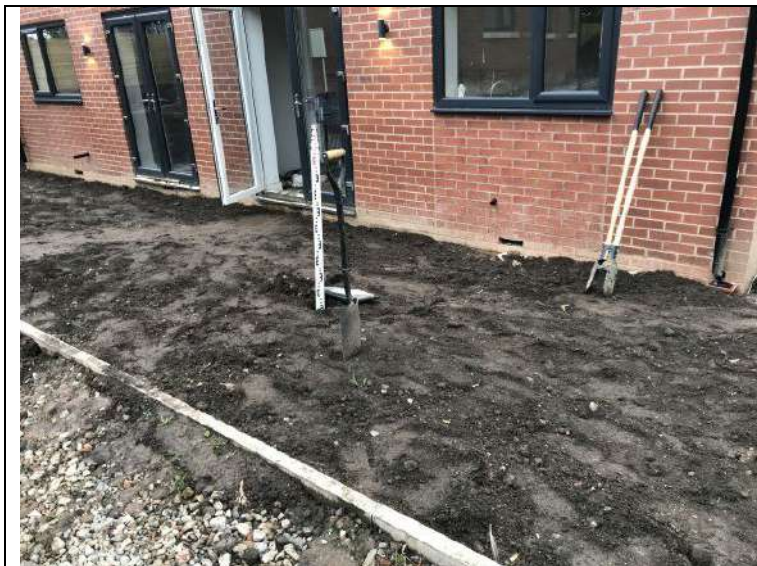
Photograph 4: View of rear garden of Plot 80.
