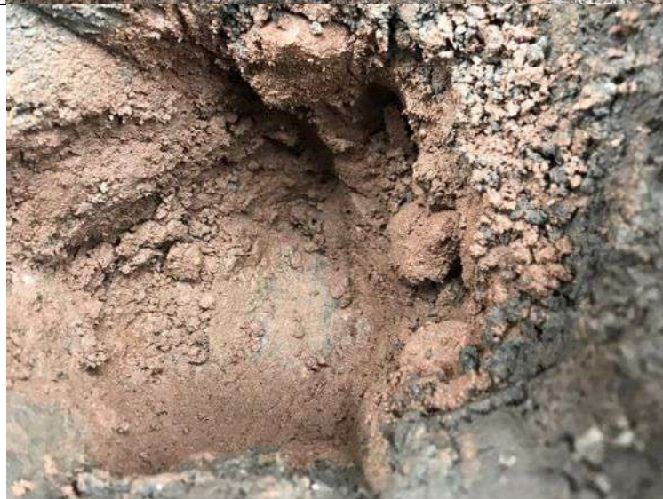
Photograph 2: View of capping layer excavation in front garden of Plot 6. Geotextile membrane present at the base.
