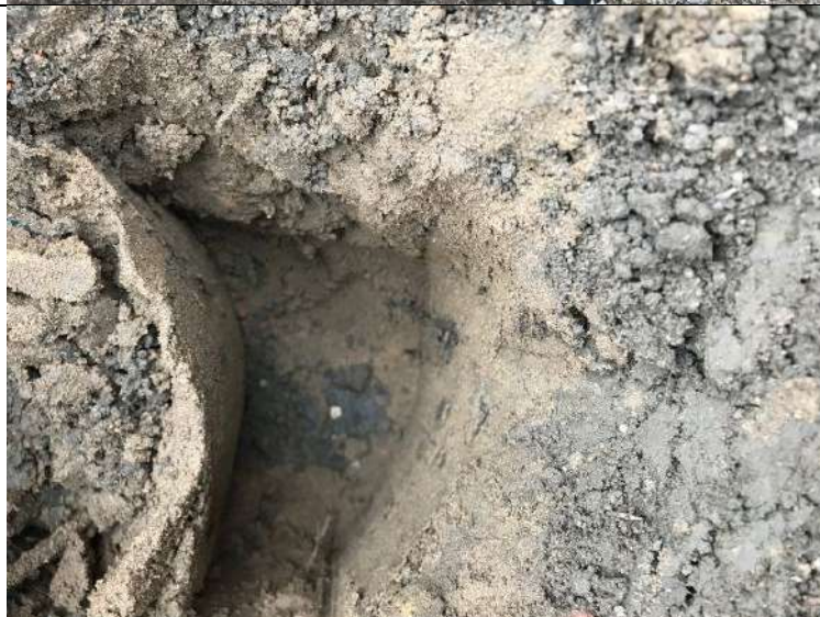
Photograph 2: View of capping layer excavation in front garden of Plot 78. Geotextile membrane present at the base.
