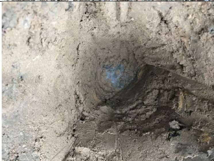
Photograph 2: View of capping layer excavation in front garden of Plot 84. Geotextile membrane present at the base.
