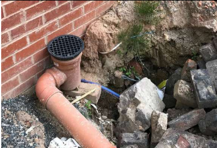
Photograph 1: Evidence of barrier pipe installed onsite.
