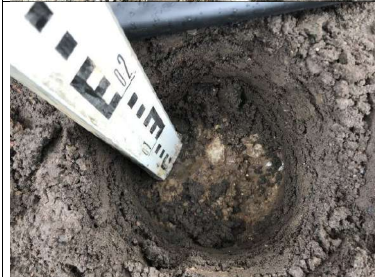
Photograph 5: View of capping layer excavation in rear garden of Plot 80. Natural clay at the base.
