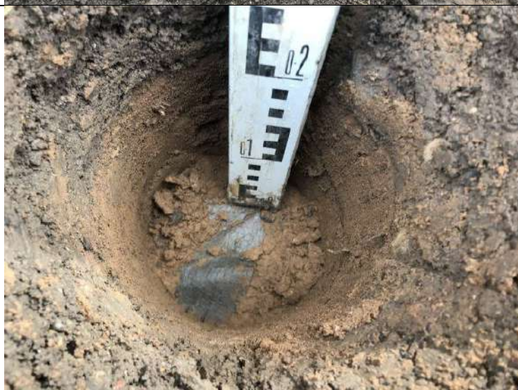
Photograph 2: View of capping layer excavation in front garden of Plot 2. Geotextile membrane present at the base.
