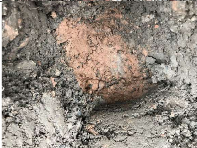
Photograph 2: View of capping layer excavation in front garden of Plot 5. Geotextile membrane present at the base.
