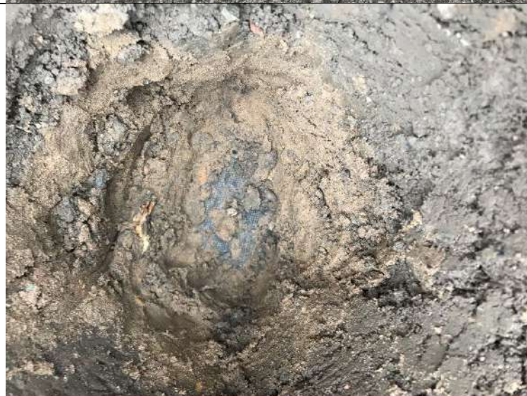
Photograph 2: View of capping layer excavation in front garden of Plot 76. Geotextile membrane present at the base.
