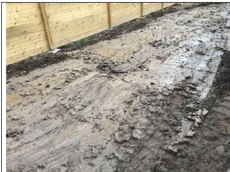
Photograph 7: Evidence of made ground removed down to natural clay at the rear of Plots 1-2 and 74.
