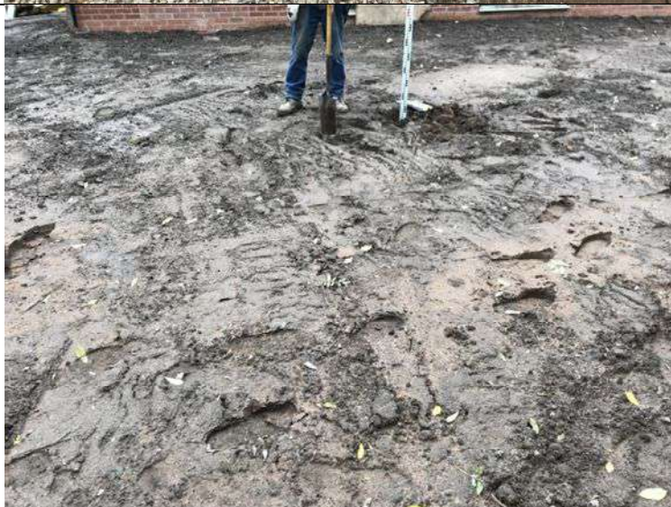
Photograph 2: View of rear garden of Plot 1.
