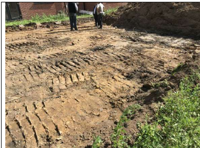
Photograph 7: Evidence of made ground removed down to natural clay.
