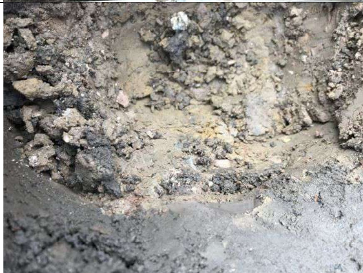
Photograph 2: View of capping layer excavation in front garden of Plot 3. Natural clay at the base.
