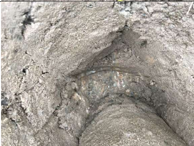
Photograph 3: View of capping layer excavation in rear garden of Plot 1. Natural clay at the base.
