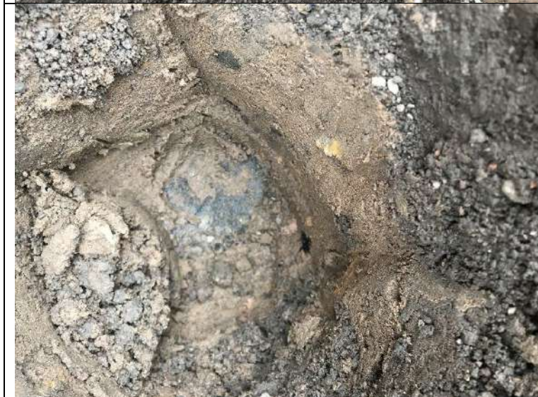
Photograph 2: View of capping layer excavation in front garden of Plot 74. Geotextile membrane present at the base.
