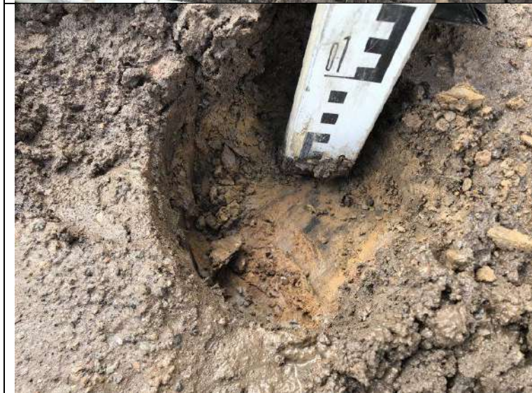
Photograph 2: View of capping layer excavation in front garden of Plot 4. Natural clay at the base.
