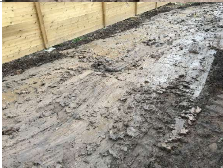
Photograph 5: Evidence of made ground removed down to natural clay to the rear of Plots 1-2 and 74.
