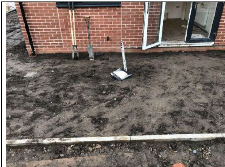
Photograph 4: View of rear garden of Plot 82.
