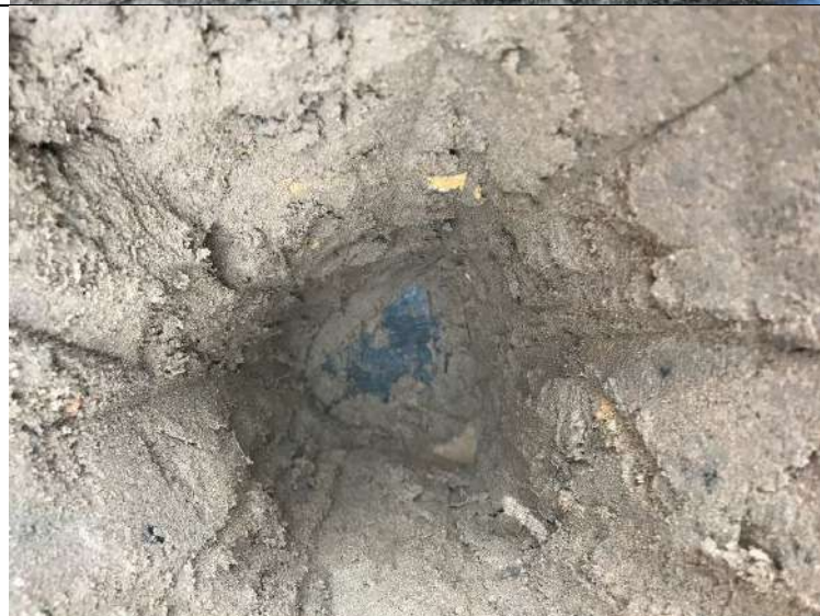
Photograph 2: View of capping layer excavation in front garden of Plot 82. Geotextile membrane present at the base.
