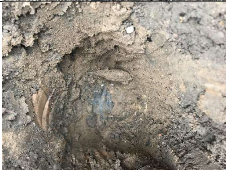
Photograph 2: View of capping layer excavation in front garden of Plot 80. Geotextile membrane present at the base.
