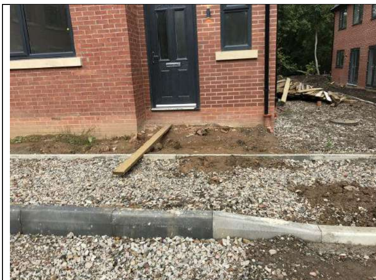
Photograph 1: View of front of Plot 1 – No garden present, all paving to be installed.
