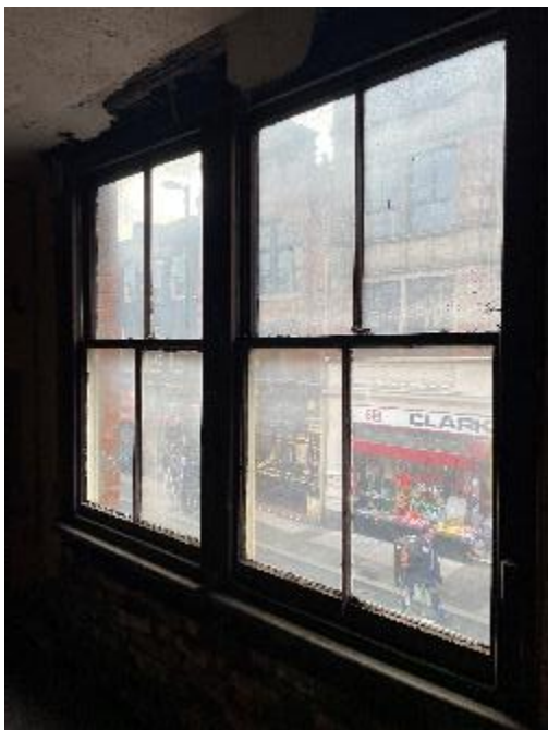
Figure 34: The two 19 th century sash windows.
