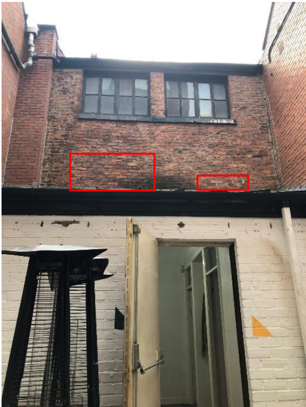
Figure 47: The rear elevation as viewed from the yard, showing the c1992 extension and blocked first floor window/taking-in door (outlined).
