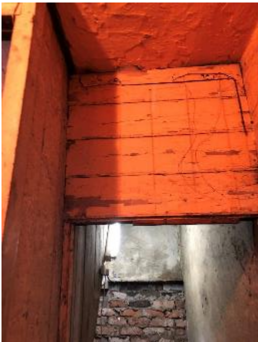
Figure 41: Simple T&G above the doorway to the small box room as seen from landing.
