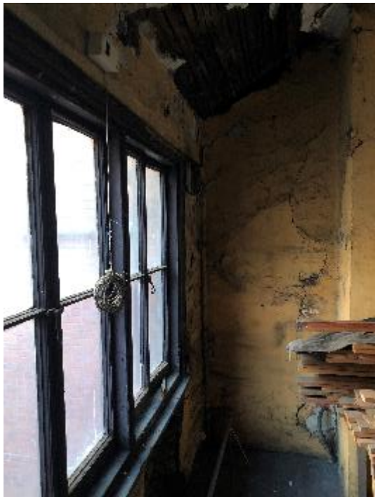
Figure 45: The 19 th century casements to the north-east elevation. The walls show evidence of originally being painted brick, with a thin layer of later plaster applied over.
