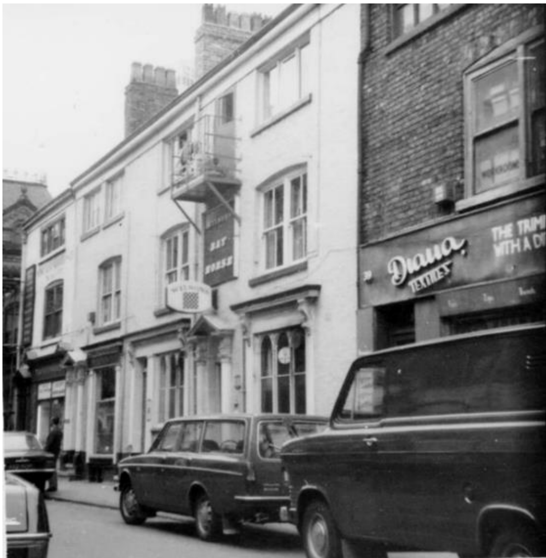
Figure 12a: A view looking west along Thomas Street towards No. 33 in 1971, showing the buildings to the left of No. 31 being demolished. (Source: Historic England)
