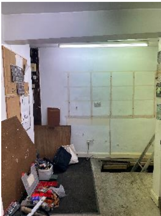
Figure 29: Looking west along the rear ground floor room, showing the floor opening leading to the basement.
