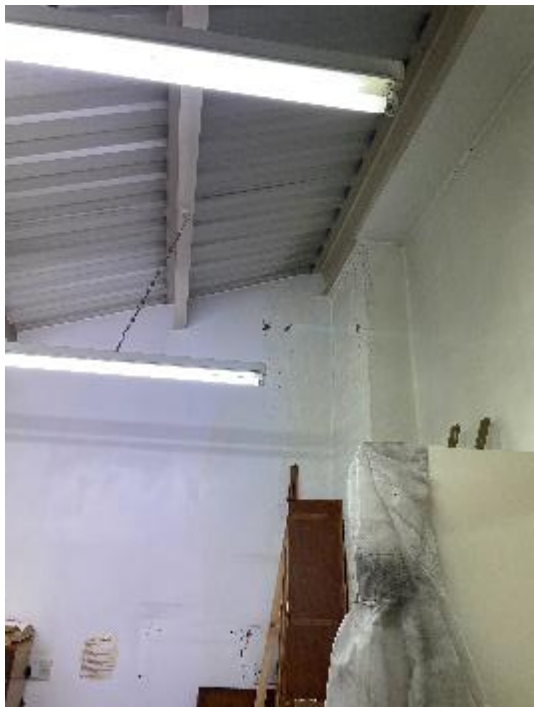
Figure 30: The c1992 rear extension.
