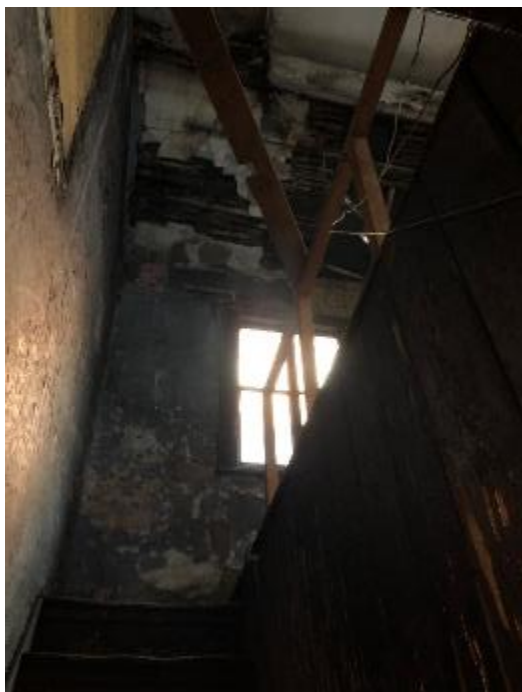
Figure 42: Looking up the original 18th century stairs into the second storey former loom shop.
