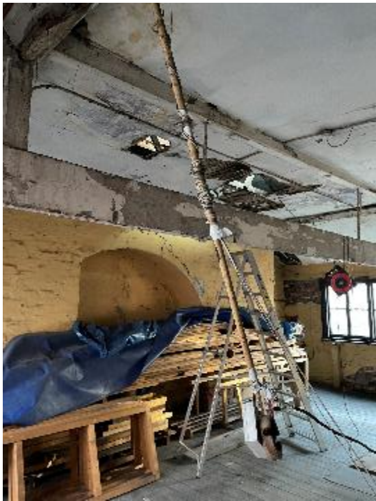
Figure 46: Looking towards the eastern side of the second floor, showing the partially exposed roof structure, original lath and plaster lowered ceiling and the two original chimney breasts (openings since filled).
