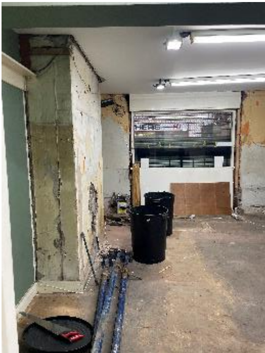
Figure 27: Looking south-west into the front room from the rear of the ground floor, showing one of two original chimney breasts.
