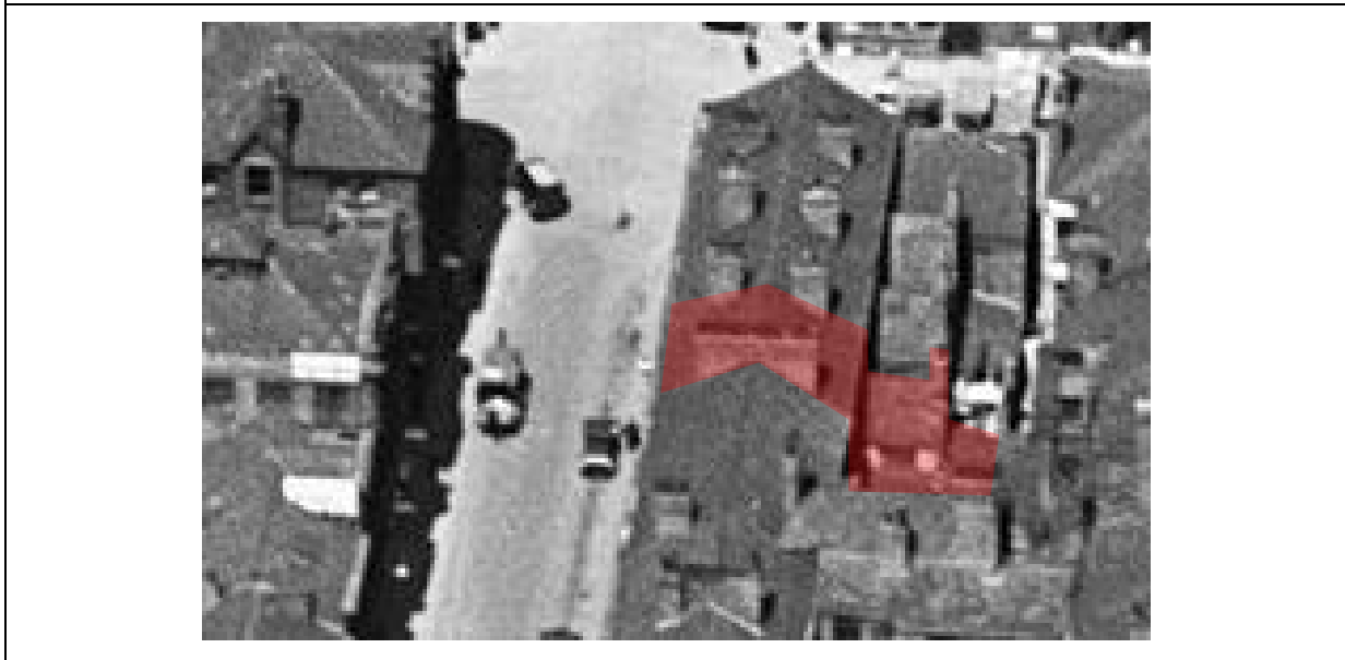
Figures 13a: An aerial view looking west across the site in 1932, showing the original, wide chimney stack to No. 33 (now removed) and original two-storey and one-storey outriggers/extensions to the rear of the site. (Source: Britain From Above)
