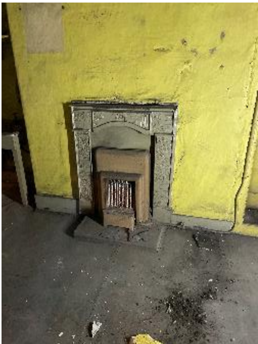
Figure 40: A mock-up of a fire surround, created in the c1950s by using pieces of painted anaglypta wallpaper pasted onto timber.
