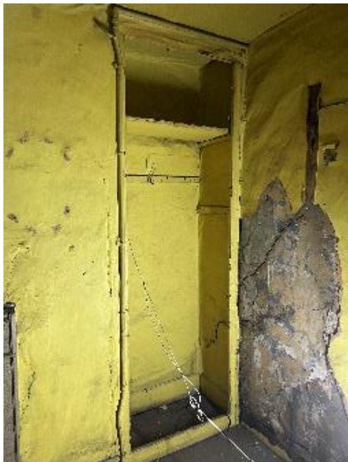
Figure 39: Remains of an original/early timber alcove cupboard in the second room.
