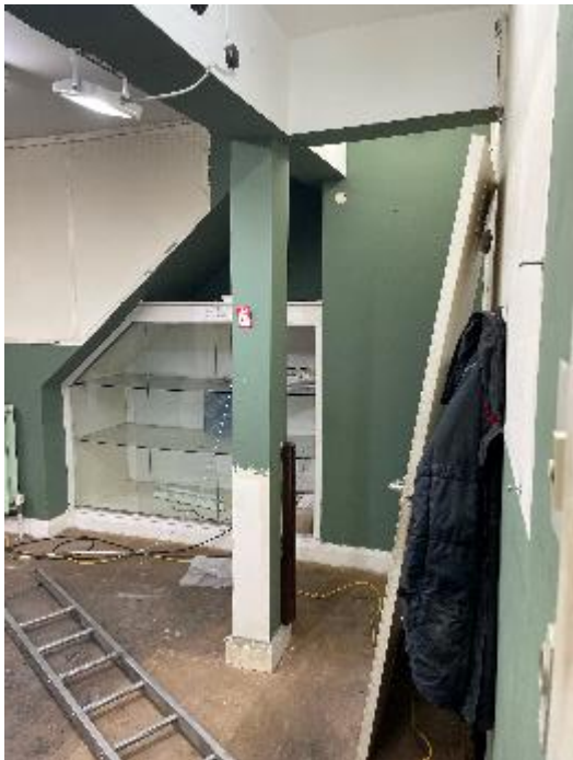
Figure 28: The modern shop display unit beneath the main staircase and locations of original walls which have since been removed.
