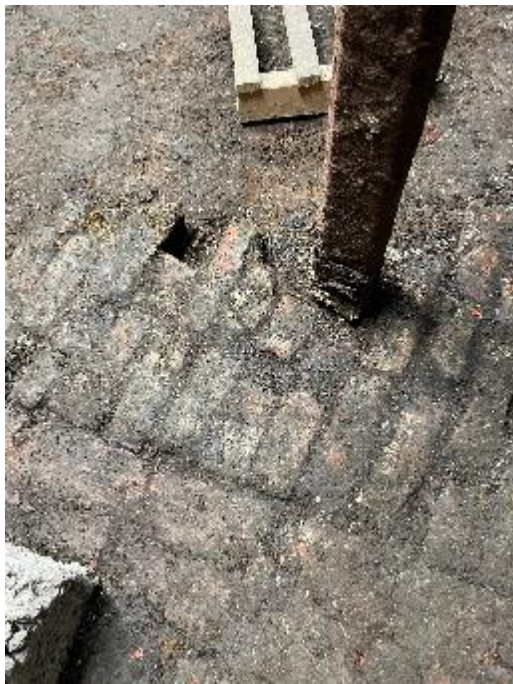
Figure 26: An example of the original red brick floor to the northern half of the basement.
