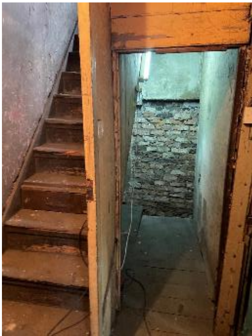
Figure 37: Looking towards the original second floor staircase/enclosure and rear box room, showing a slight floor ramp and filled-in former taking-in door from the rear yard.
