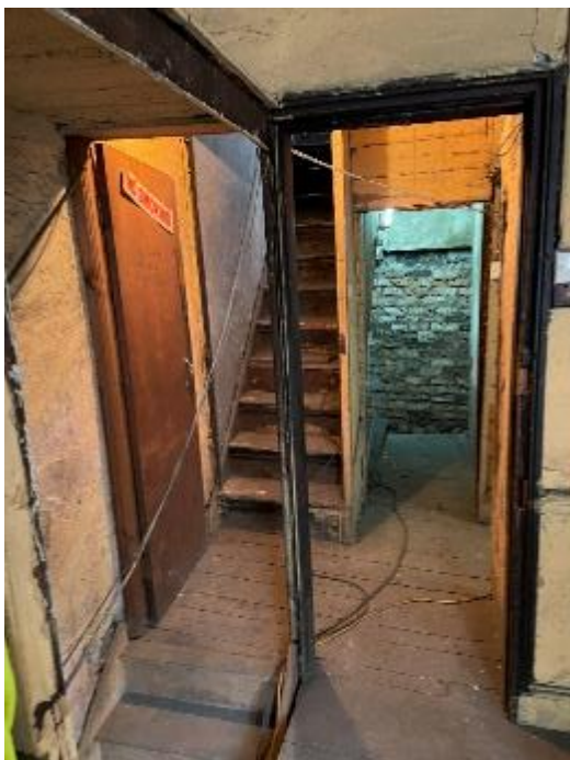
Figure 31: Looking from the main front room into the small landing, with staircase to second floor to the left, and entrance into small box room to its right hand side.
