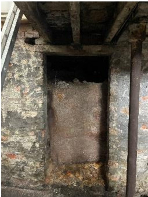
Figure 25: The now blocked doorway into the original rear outrigger to the northern corner of the basement.
