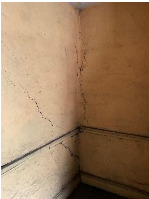
Figure 33: A detail of the original dado and skirting along with 18 th century surviving wall plaster.
