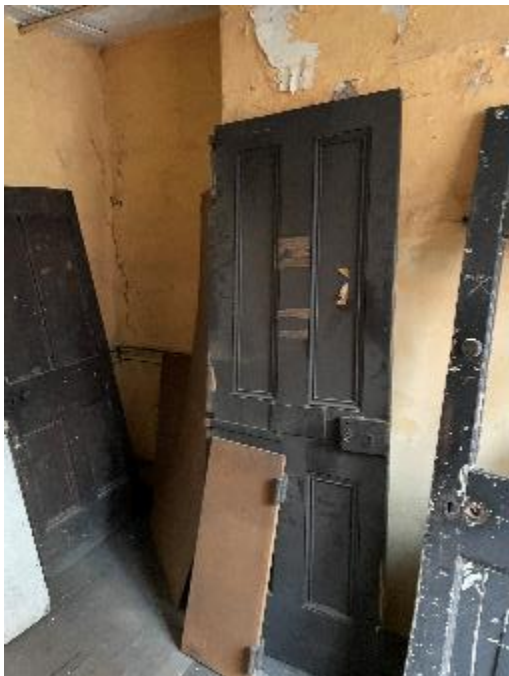
Figure 36: A collection of three 18 th and 19 th century doors from the first floor temporarily removed.
