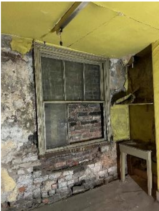
Figure 38: Looking into the second rear room, showing the remains of a 19 th century tripartite sash window and late-19 th /early-20 th century sink to alcove.
