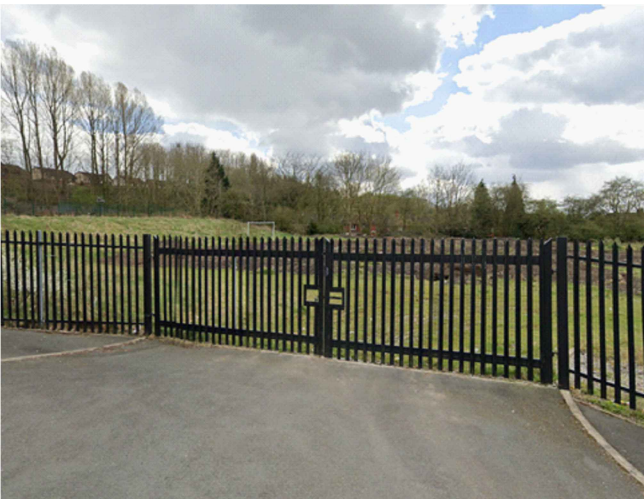
1. Location of existing double gates into the site
