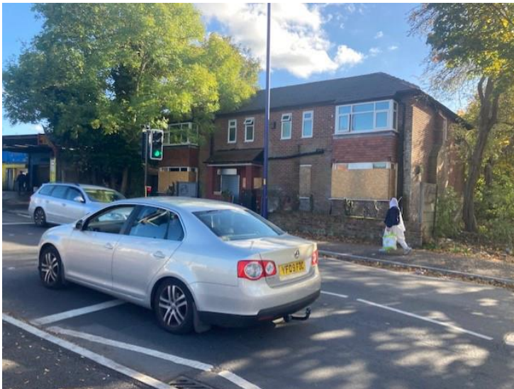
View of the front from Moston Lane
