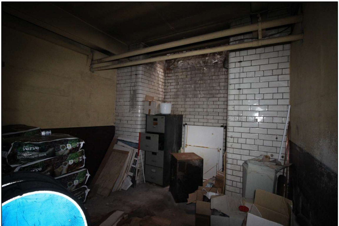
Plate 14: The central room to the basement, detailing the white glazed bricks to the northern wall
