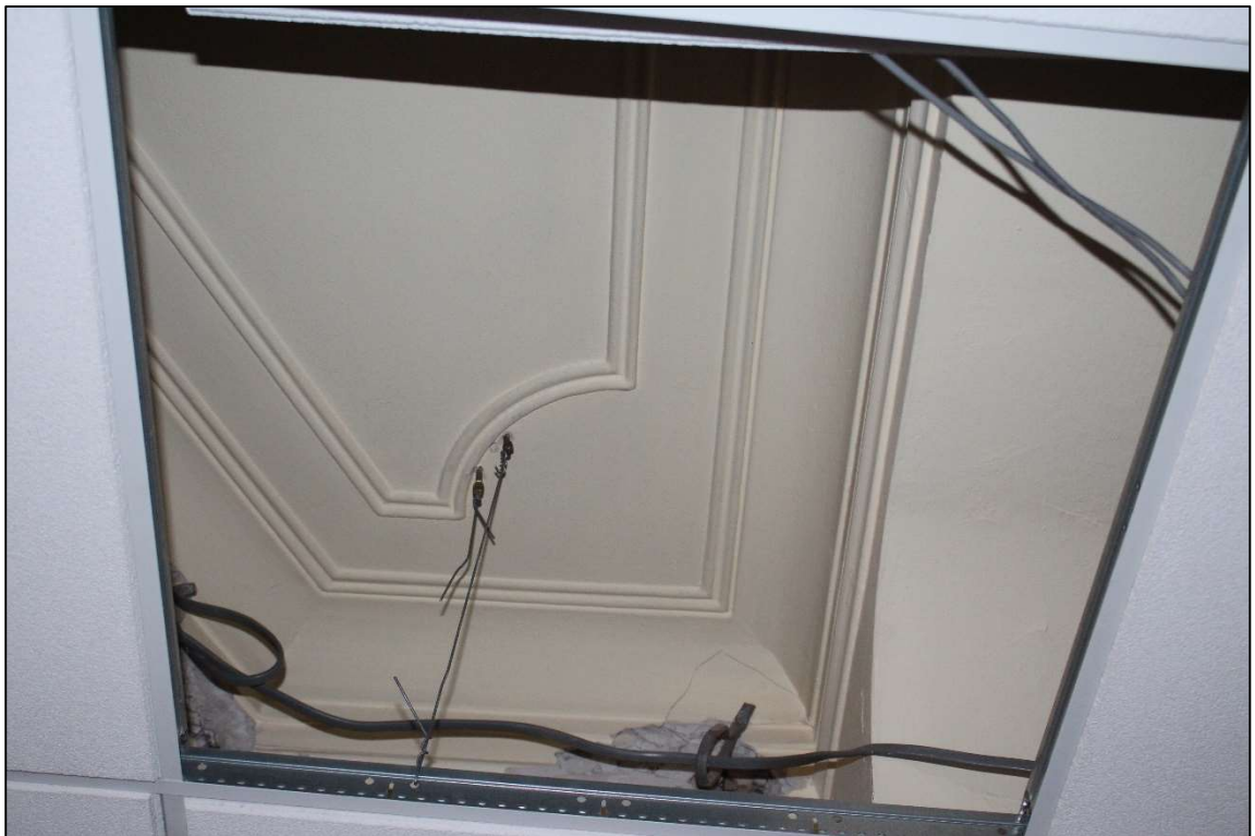
Plate 11: The original coffer ceiling to one of the rooms on the fourth floor
