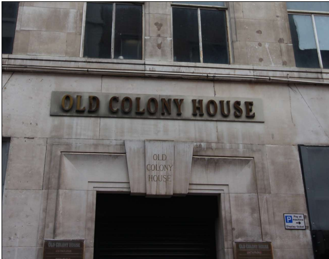
Plate 3: Detail of the Art Deco keystone to the central doorway within the northern elevation
