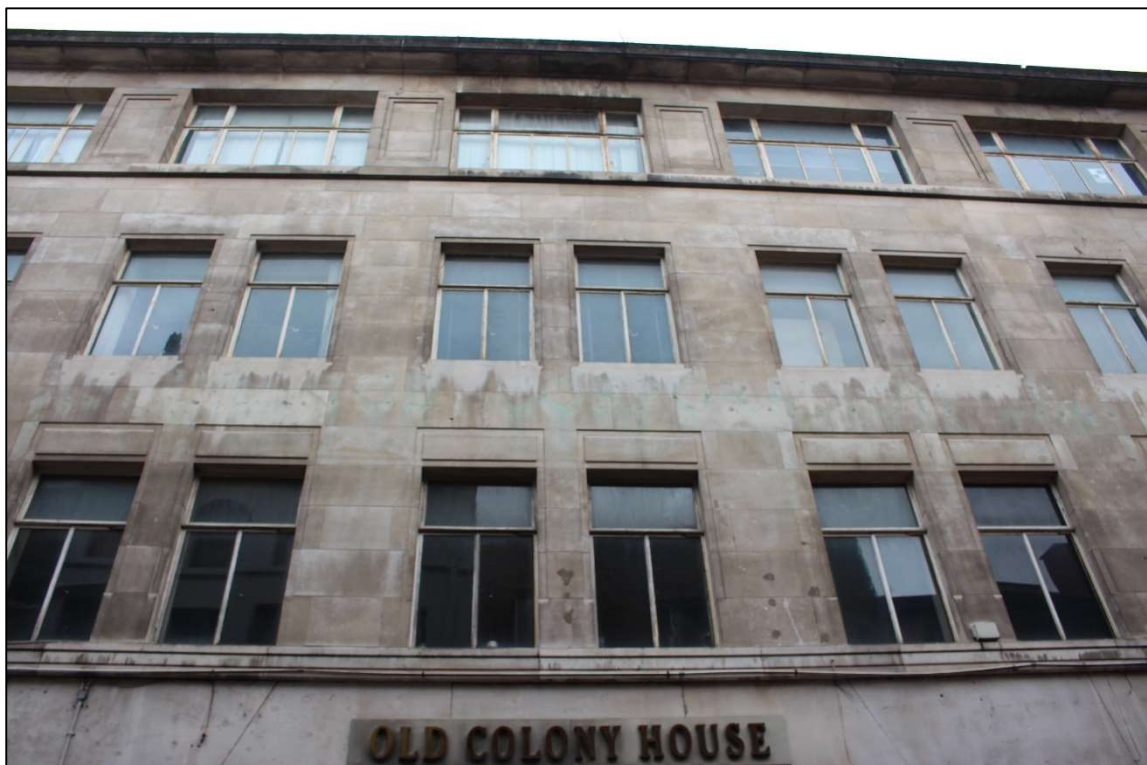
Plate 4: Detail of the upper floor apertures to the northern elevation
