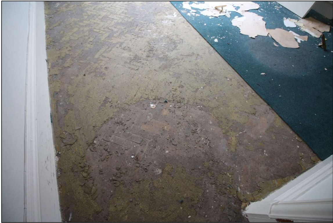
Plate 12: The timber herringbone floor below the modern carpet floor on the fifth floor
