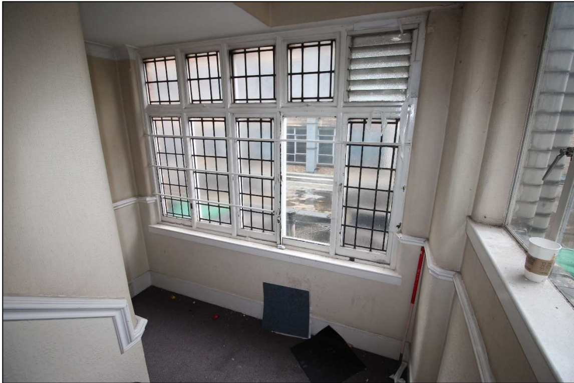
Plate 9: The original steel casement window to the fourth floor landing
