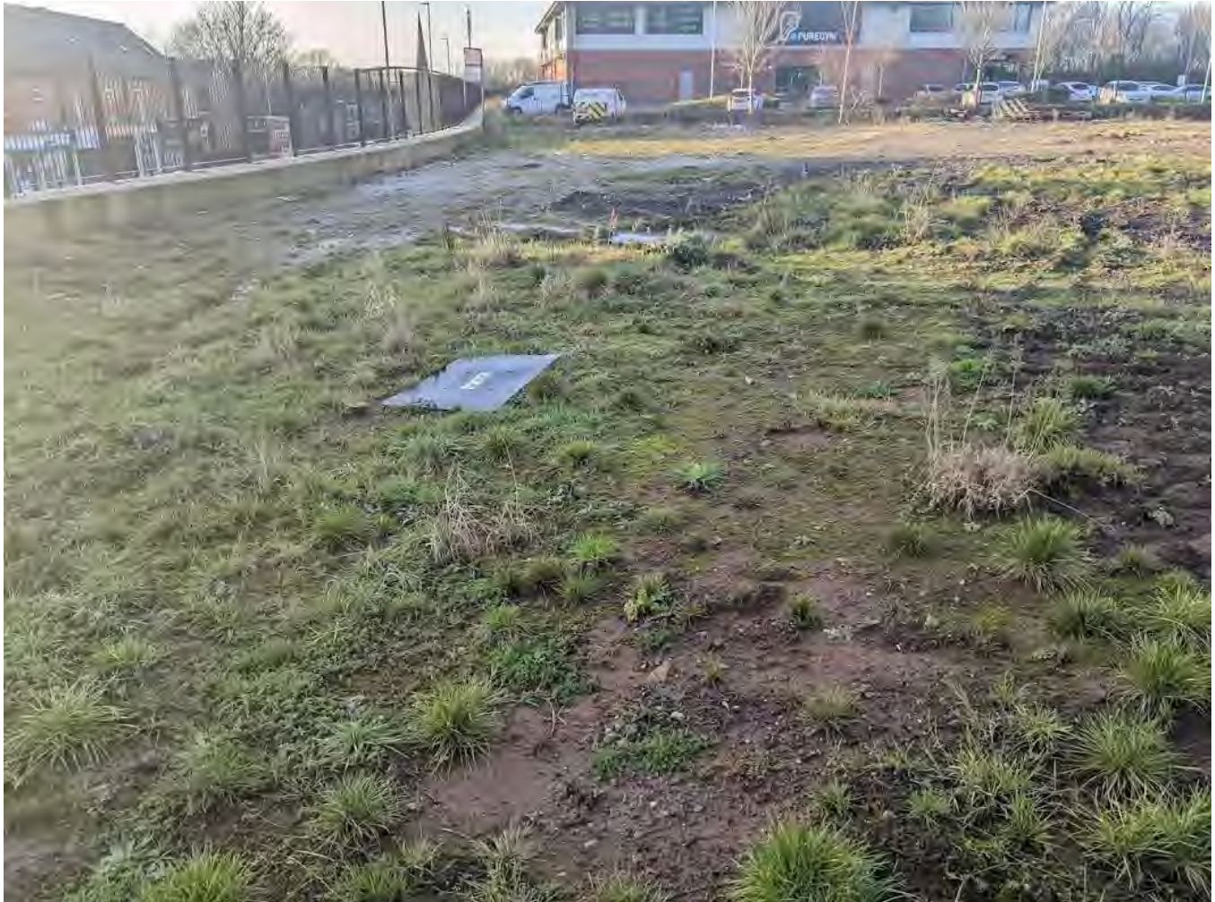
C4 – Southern boundary and retaining wall (looking west)
