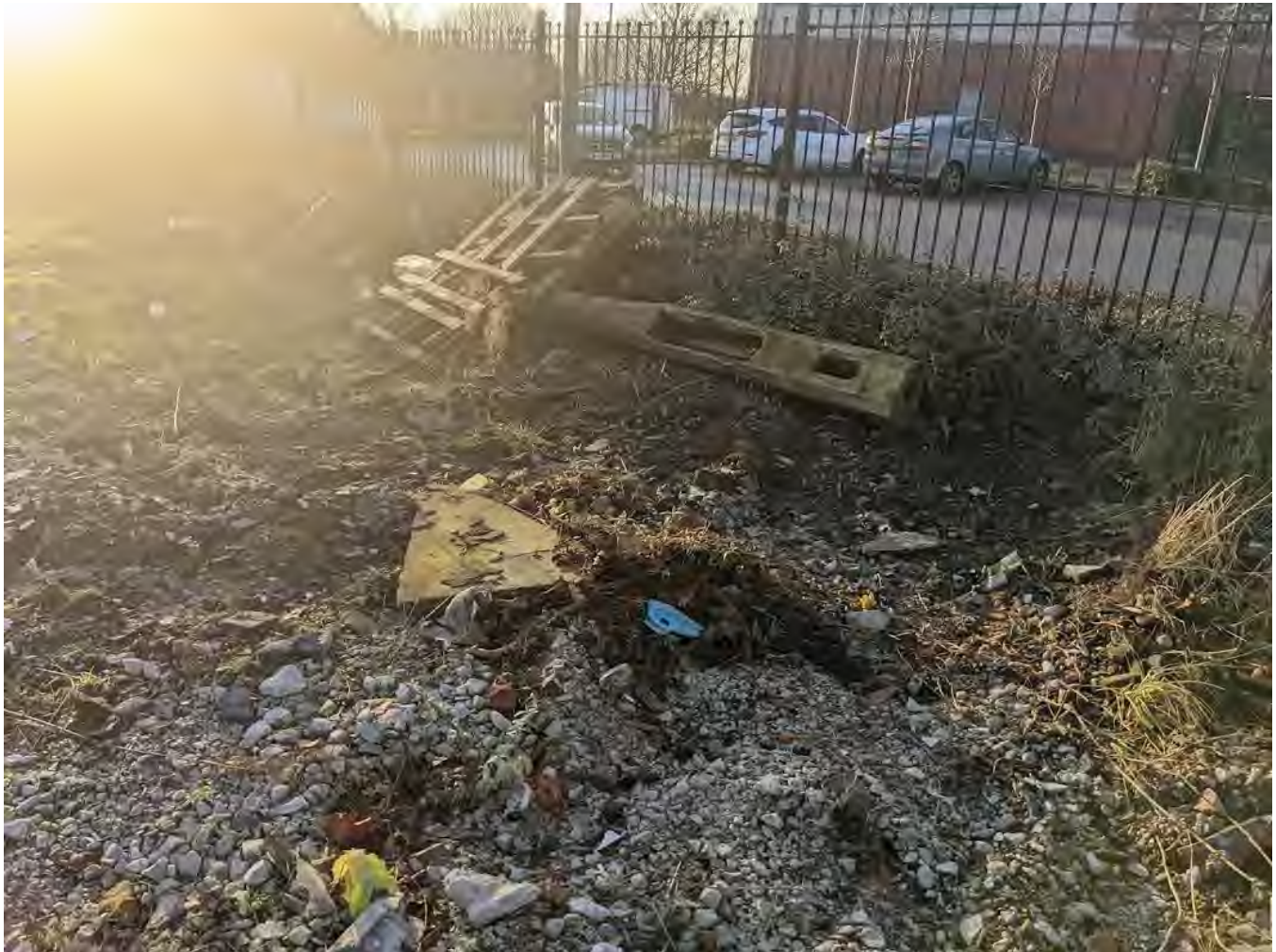
C6 – Possible signs of fly tipping/waste at northwest corner (looking southwest)
