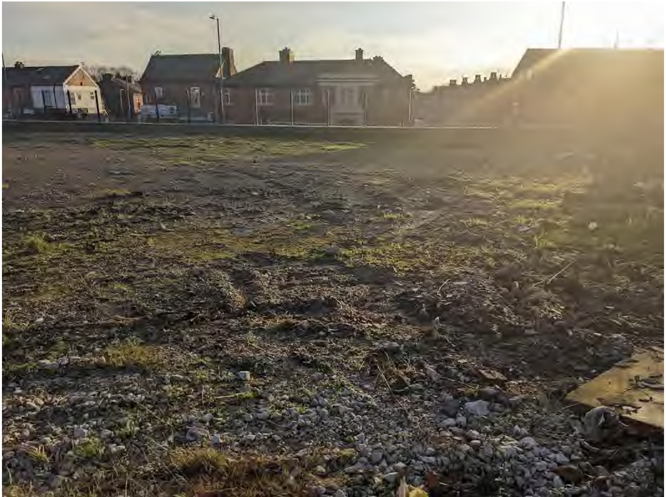
C5 – Southern boundary and retaining wall (looking south)
