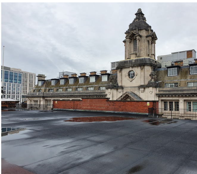
Image 02: Churchgate Roof Towards Oxford Road
