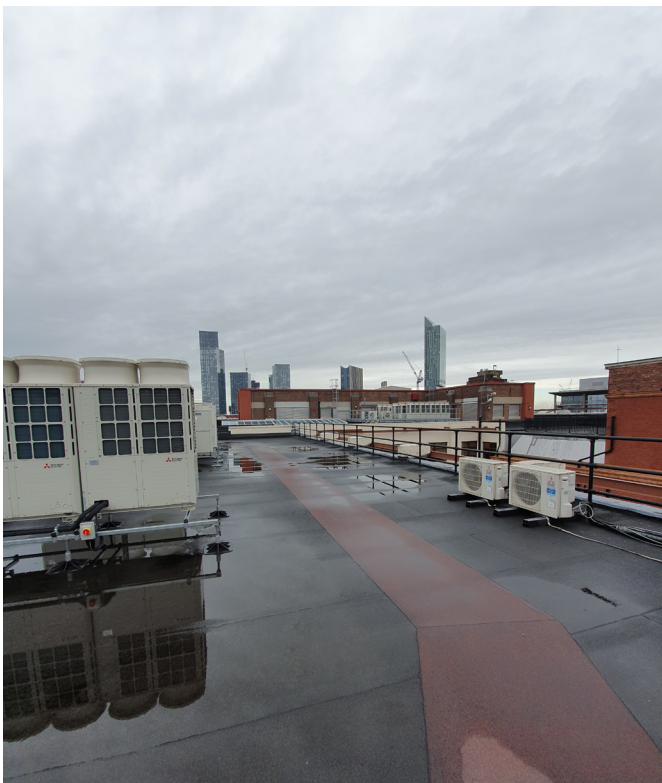
Image 01: Churchgate Roof Towards Lee Roof
