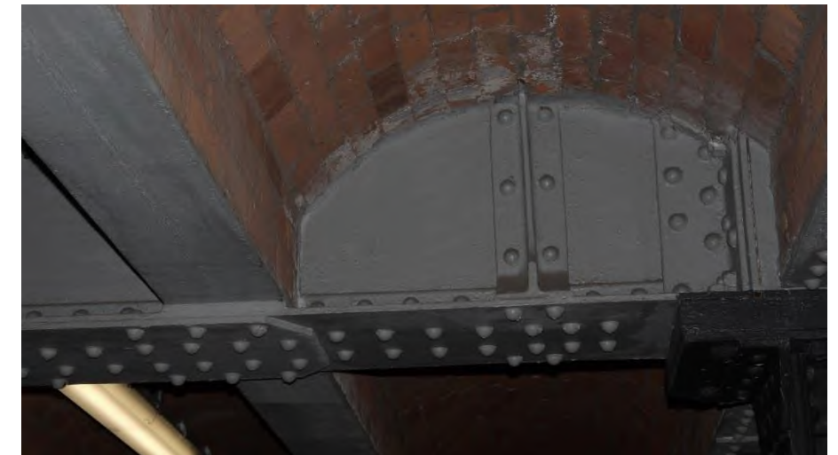
Figure 4.1: Web stiffeners / angle connection
