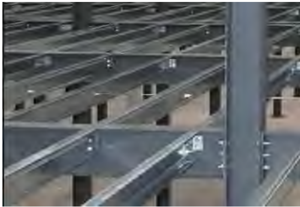
Figure 7.4: Lightweight floor support on hot rolled steel
