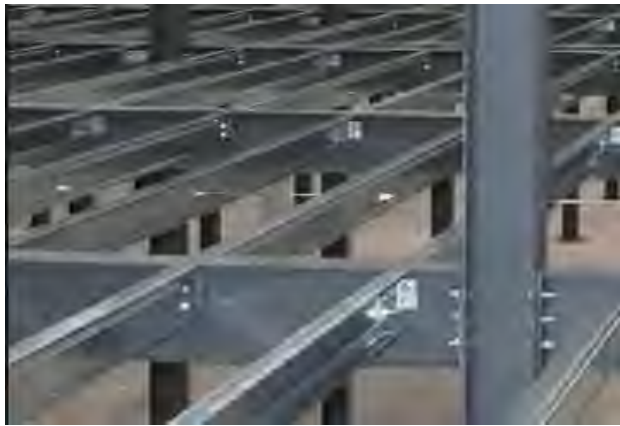
Figure 7.4: Lightweight floor support on hot rolled steel
