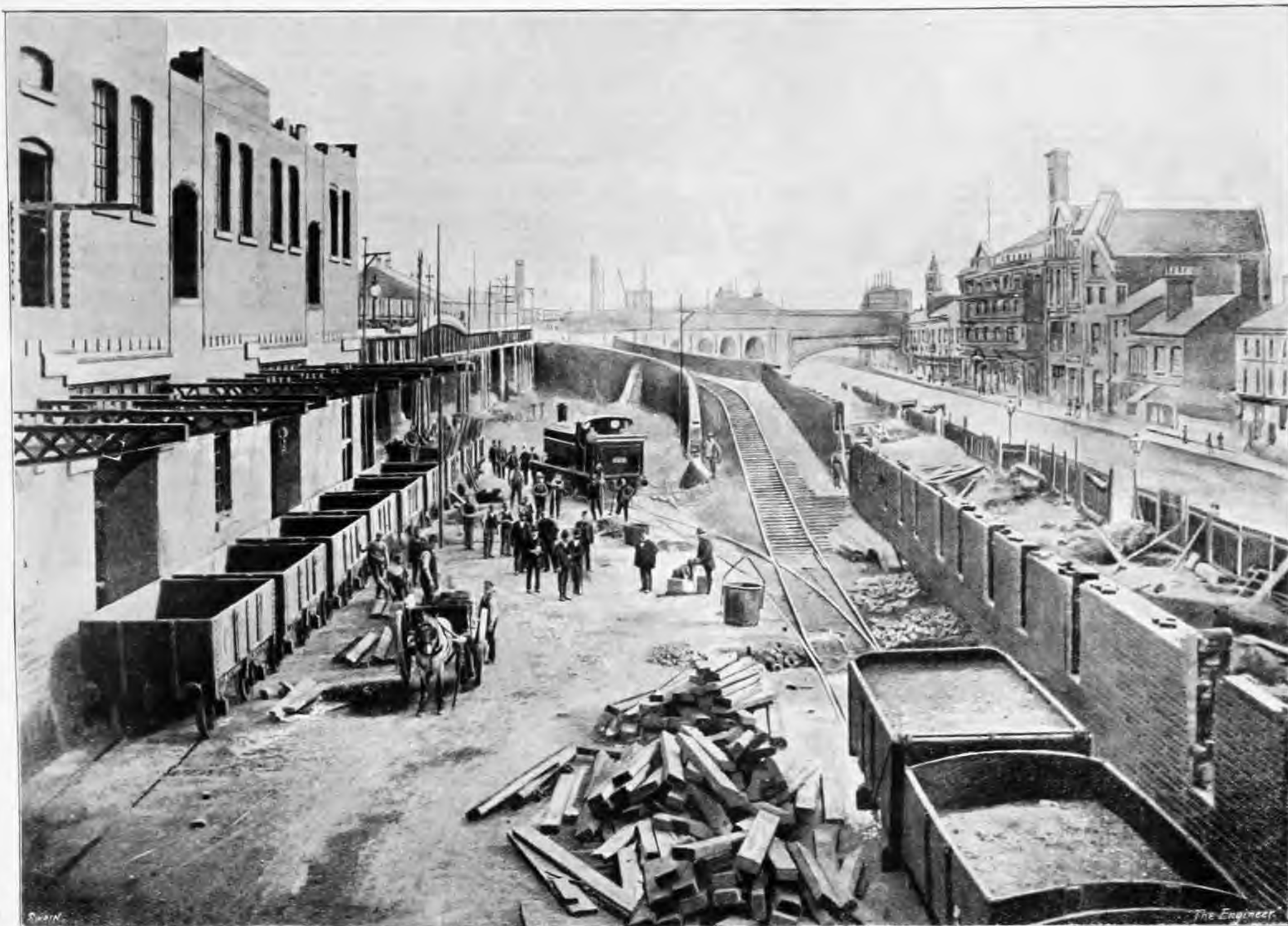
WESTERN INCLINED PLANE TO LOW-LEVEL YARD
