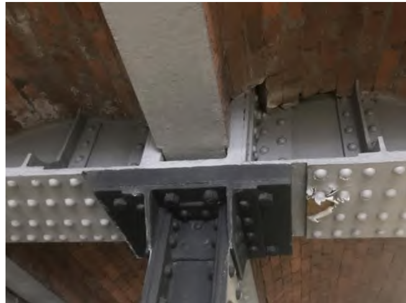
Figure 4.0: Connection junction at floor
