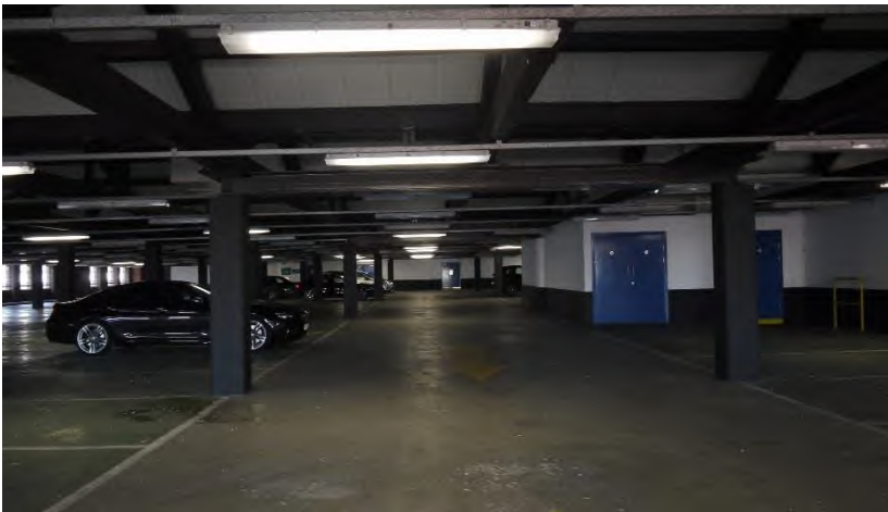
Figure 3.3: Column removal installation of transfer beams
