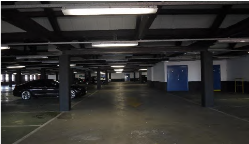
Figure 3.3: Column removal installation of transfer beams
