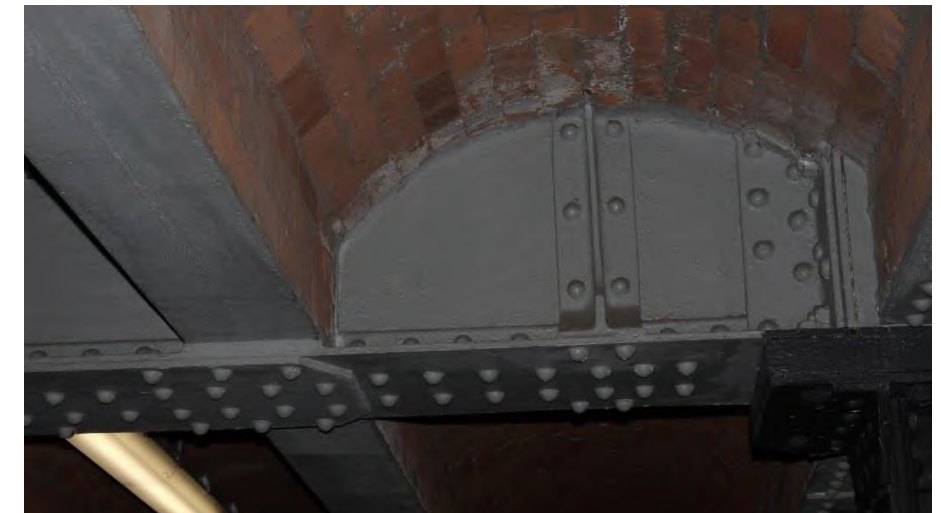
Figure 4.1: Web stiffeners / angle connection
