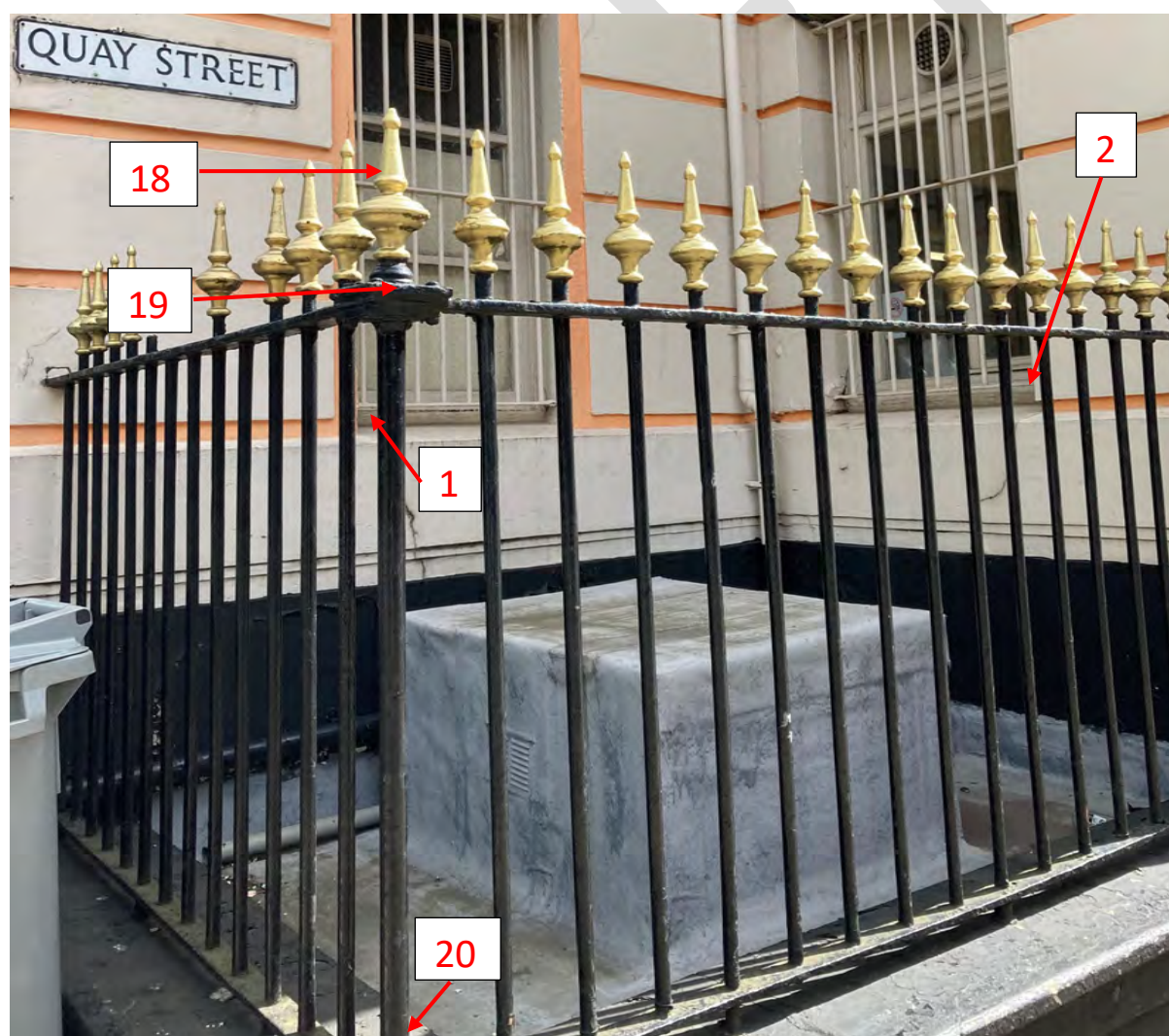
Figure 5: sample locations 1, 2 (windows W2-F and W3-F) & 18 – 20 (railings)
