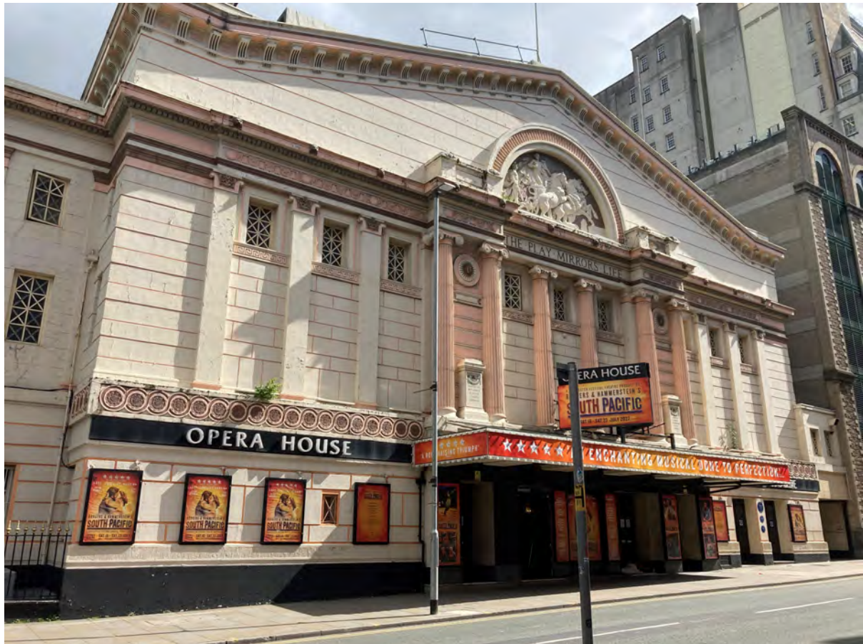
Figure 1: The Opera House façade facing the road
