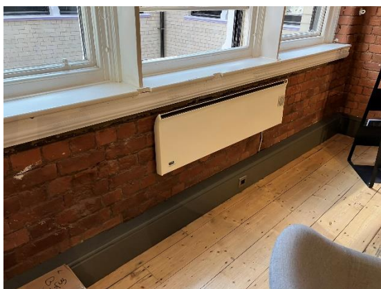
Photo 11: Typical modern panel radiator
