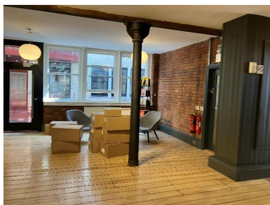
Photo 4: View towards the central Atrium. Access to the stair core is to the right. Modern panel radiator visible beneath the window
