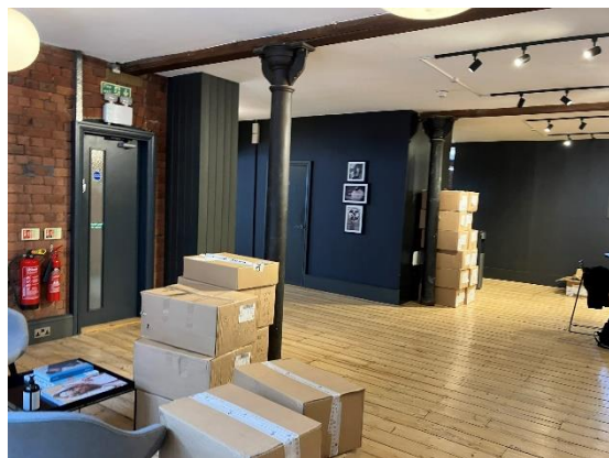
Photo 1: Looking west across Unit 05 towards the modern WC enclosure. Original cast-iron columns and timber beams are evident
