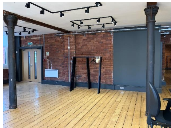
Photo 10: View towards the stair core. The modern partition enclosing the store and WC are evident against the historic brickwork.
