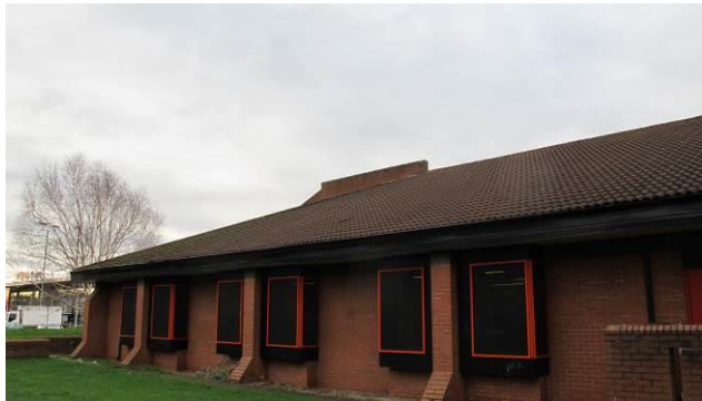
Photo 2 – side of the building showing the Windows covered in mesh
