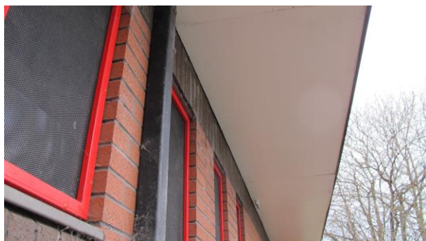
Photo 7 – underside of the cornice
