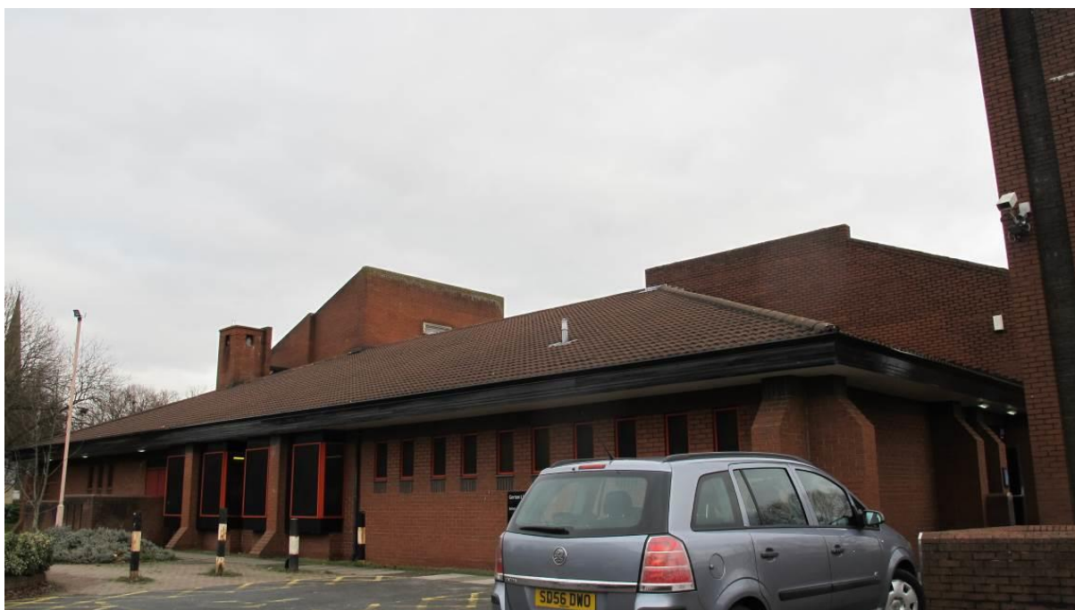
Photo 4 – structure to the roof which houses the boiler and heating equipment
