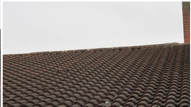
Photo 3 – overlapping concrete tiled roof
