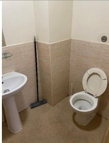
Photograph 19, First Floor, Typical WC
