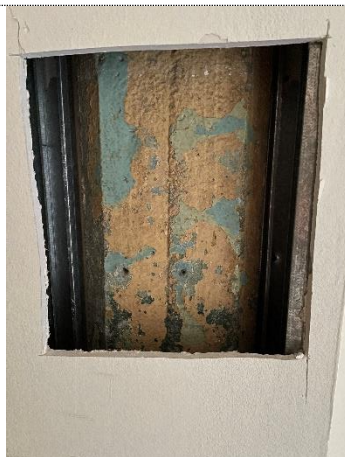
Photograph 41, Fourth Floor, Typical concrete column boxed in
