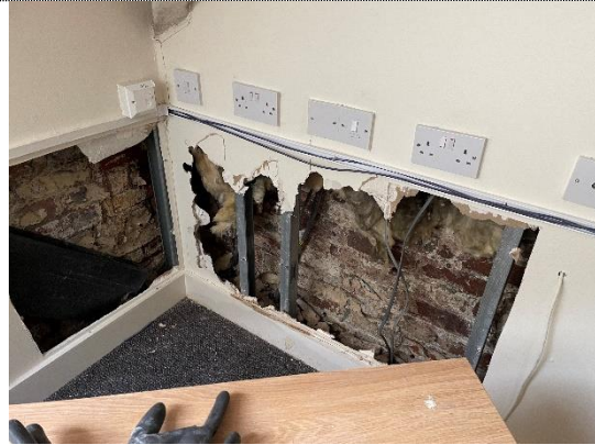
Photograph 44, Fifth Floor, Typical drylining to external walls
