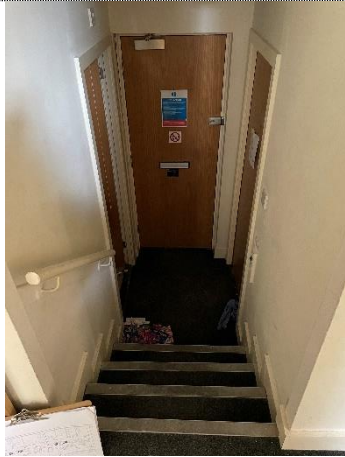
Photograph 43, Fifth Floor, Typical internal corridor
