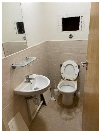
Photograph 29, Second Floor, Typical WC
