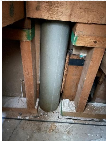
Photograph 45, Fifth Floor, Typical suspended floor
