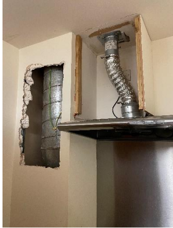
Photograph 31, Third Floor, Typical ventilation ducts boxed in
