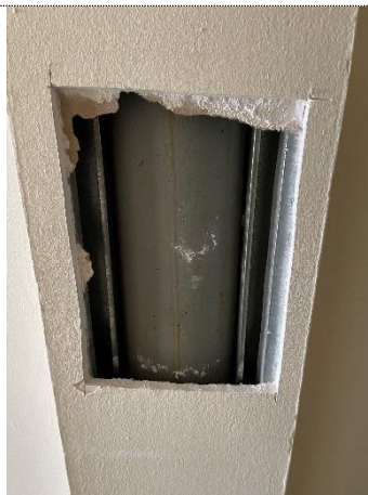
Photograph 42, Fourth Floor, Typical steel column boxed in
