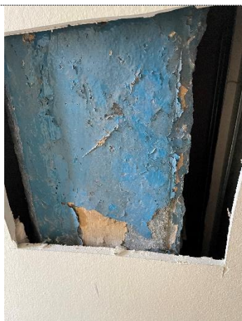
Photograph 35, Third Floor, Typical concrete column boxed in
