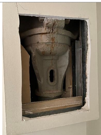
Photograph 48, Fifth Floor, Typical steel column boxed in
