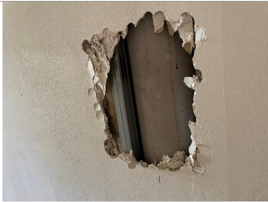
Photograph 13, Ground Floor, Typical steel column boxed in
