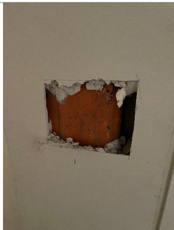
Photograph 21, First Floor, Typical concrete column boxed in
