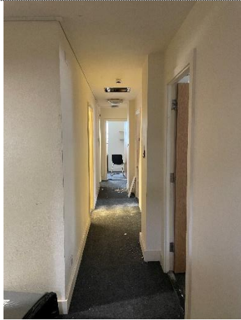
Photograph 25, Second Floor, Typical corridor inside flats
