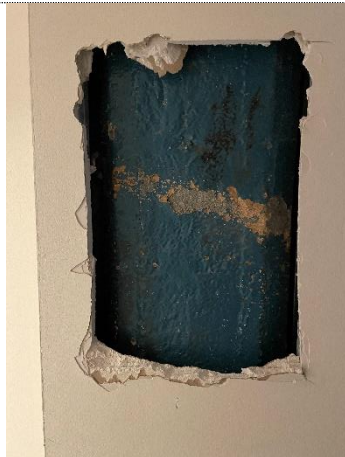
Photograph 33, Third Floor, Typical concrete column boxed in
