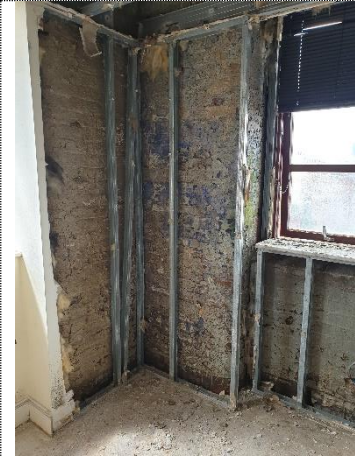
Photograph 37, Fourth Floor, Typical drylining to external walls
