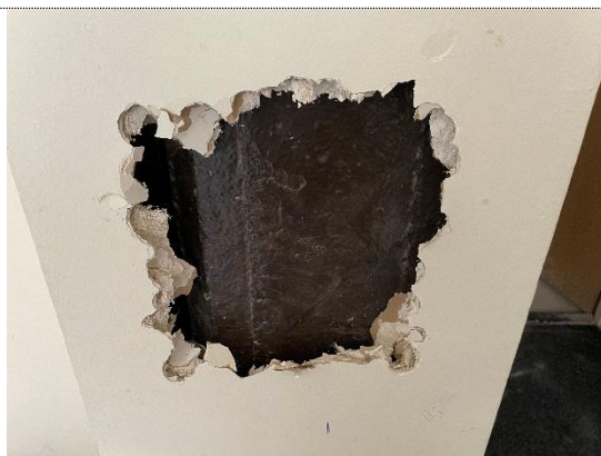
Photograph 12, Ground Floor, Typical concrete column boxed in
