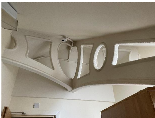
Photograph 47, Fifth Floor, Typical trusses
