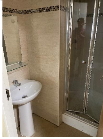
Photograph 20, First Floor, Typical Shower
