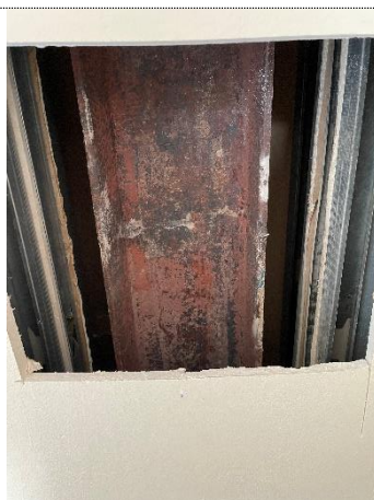
Photograph 36, Third Floor, Typical steel column boxed in
