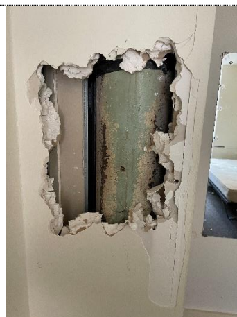
Photograph 30, Second Floor, Typical steel column boxed in
