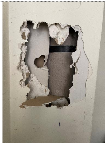
Photograph 22, First Floor, Typical steel column boxed in
