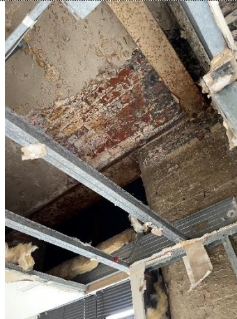
Photograph 38, Fourth Floor, Typical ceiling void
