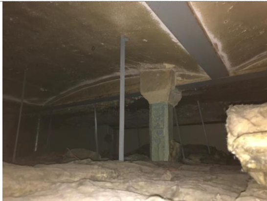
Photograph 39, Fourth Floor, Typical ceiling void
