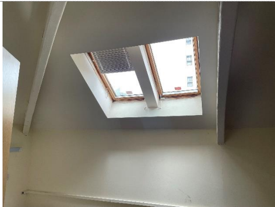
Photograph 51, Fifth Floor, Typical rooflights
