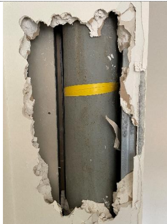
Photograph 34, Third Floor, Typical steel column boxed in
