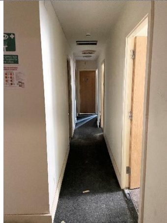
Photograph 08, Ground Floor, Typical corridor inside flats
