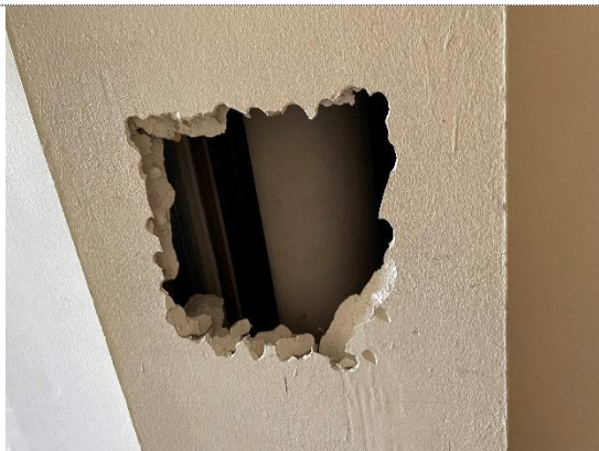
Photograph 23, First Floor, Typical steel column boxed in
