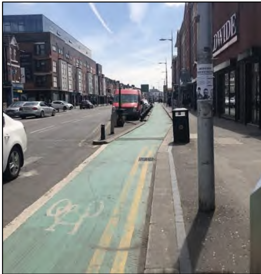
Figure 4-2 Segregated cycle lanes on Oxford Road (Oxford Road Corridor)
