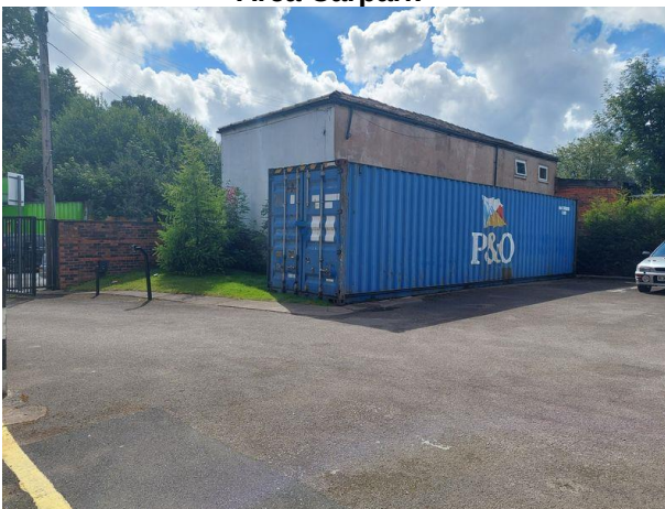
Plate 9.11: Shipping Container Situated to the South of Carpark
