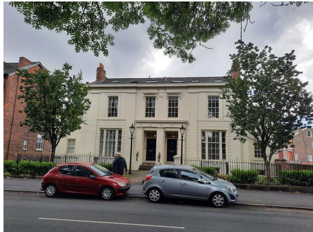
Plate 9.4: Northern Side of B2 Painted entirely white and in Good Condition
