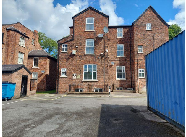
Plate 9.2: B1 With Irregular Shaped Roof and Walls
