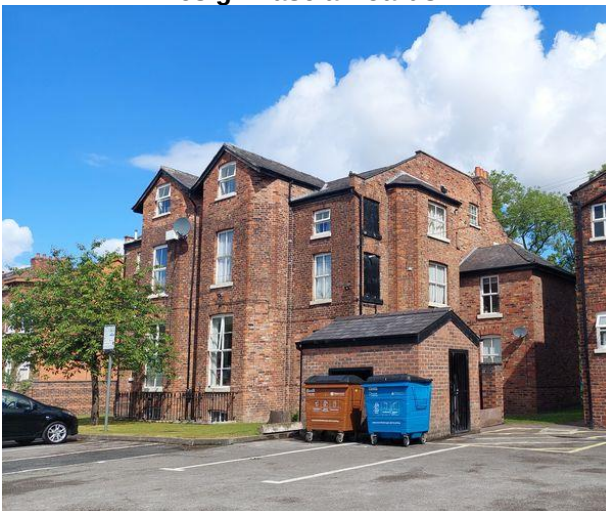
Plate 9.5: Southern Side of B2
