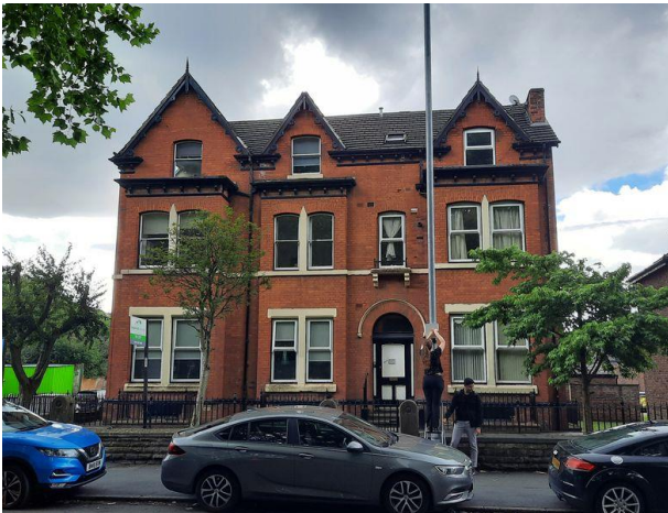
Plate 9.3: Northern Side of B1 with Ornate Design Fascia Boards
