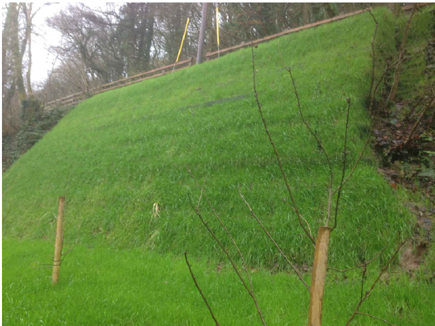
Detail 03 Soil Reinforced Wall faced with Deltalok
