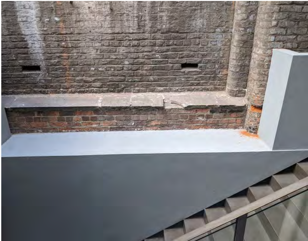
Upper ground view of stair showing existing 'boxing in' reamining from CUBE fit-out
