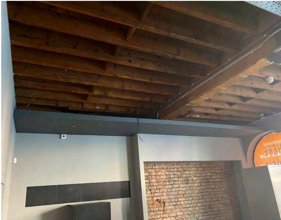
Existing view at upper ground to front section overlooking Portland Street
