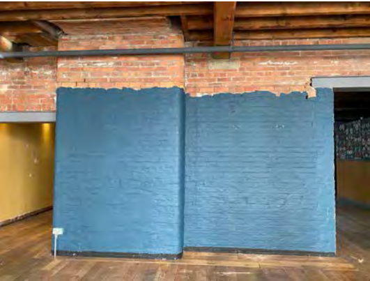
'CORE B' - paint to be removed and brickwork exposed
