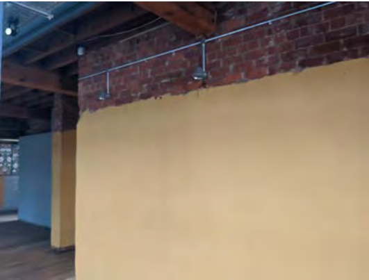
'CORE A': plastered wall to receive fabric panels, high level brickwork left exposed
