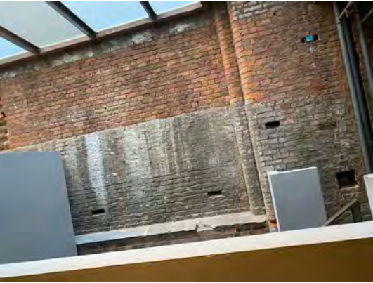
FLANK WALL 1 upper ground: brickwork exposed & lightly cleaned
