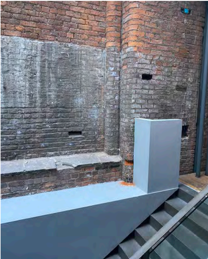
Existing view: Upper ground looking over main stair
