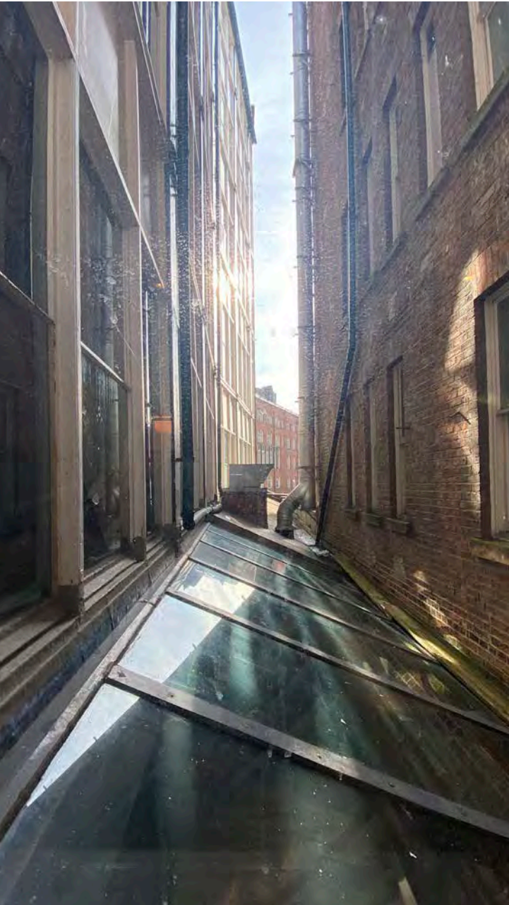
View at upper ground over lower ground rooflight
