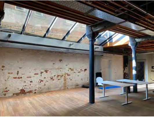
FLANK WALL 2 lower ground: paint to be removed and brickwork exposed
