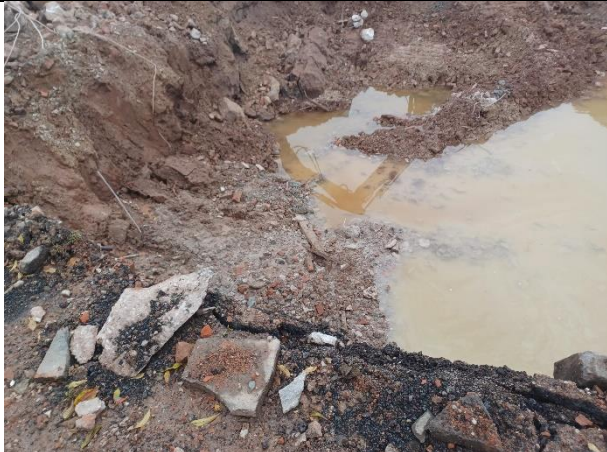
P11: Area following the full removal of the oil tank and foundation/slab.
