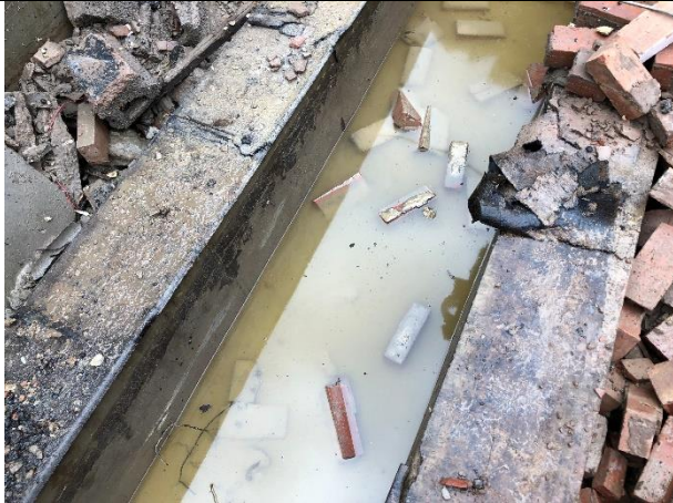
P9: Area where tank formerly sat
