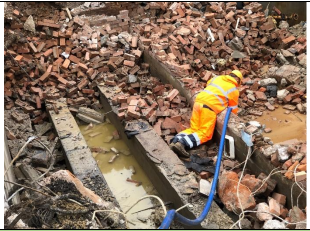
P8: Area where tank formerly sat
