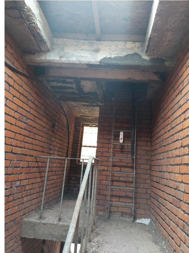
Interior of B1 (pictured above).
