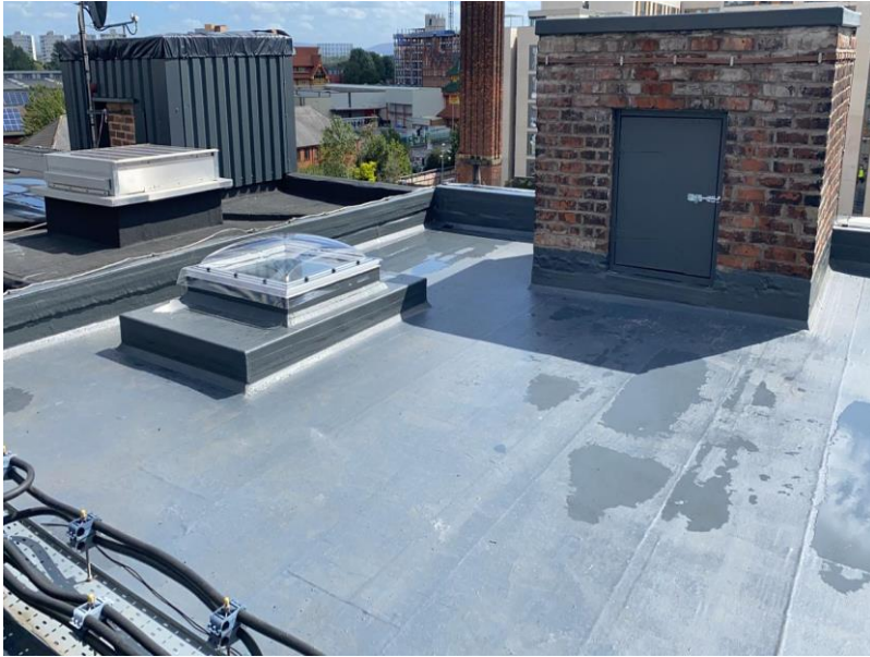
Roof of B1 taken by the client (pictured above).
