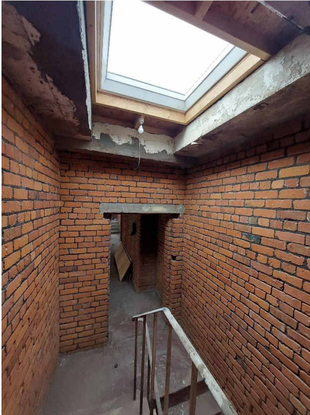
Interior of B1 (pictured above).
