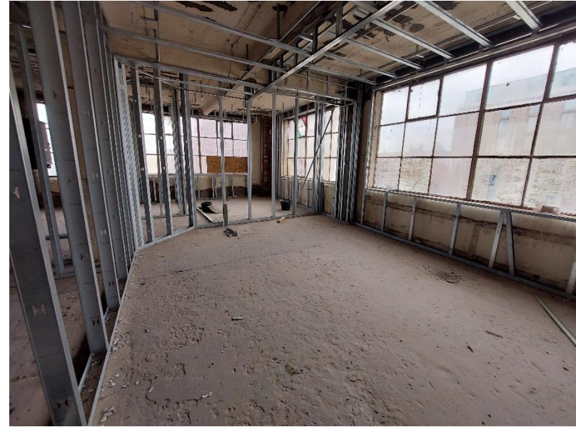
Interior of B1 (pictured above).
