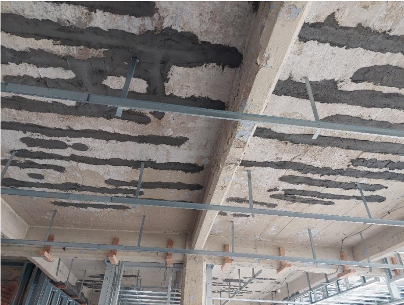
Interior of B1 (pictured above).
