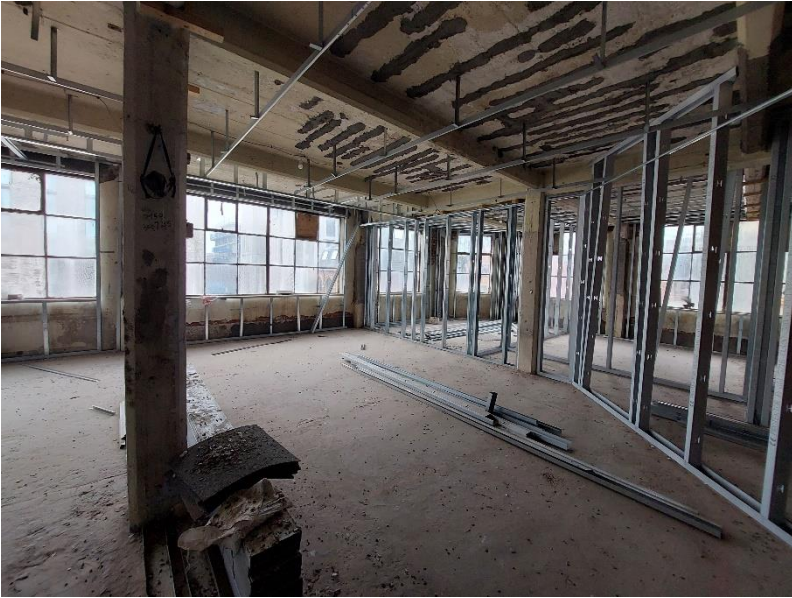
Interior of B1 (pictured above).
