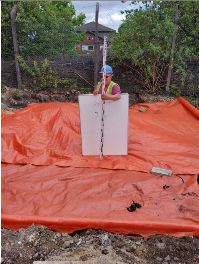
Photograph 3: Reduced level dig and membrane within rear garden of plot 24.
