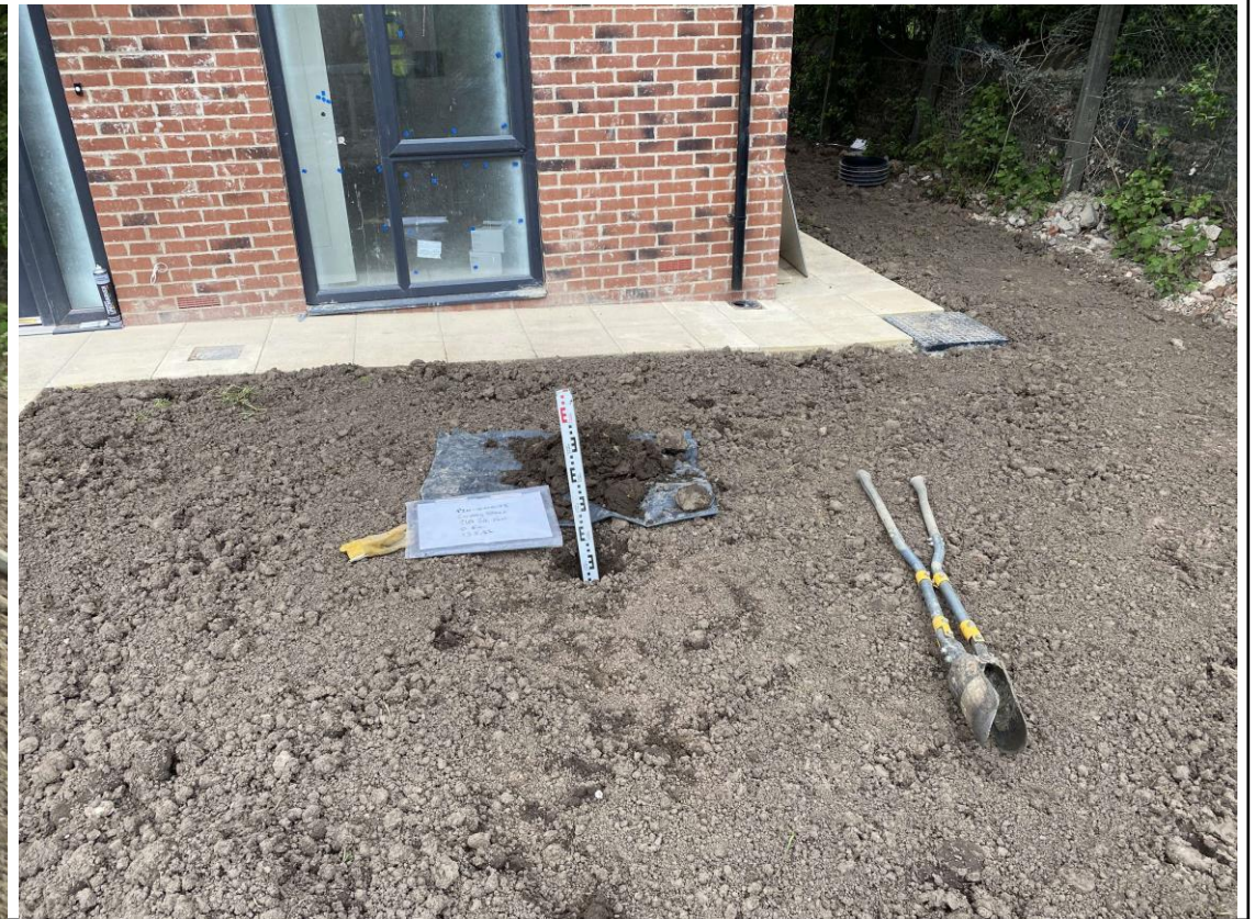
Photographs 9 and 10: Hand Dug Pit Topsoil Depth Validation – HDP19, Plot 24 Front
