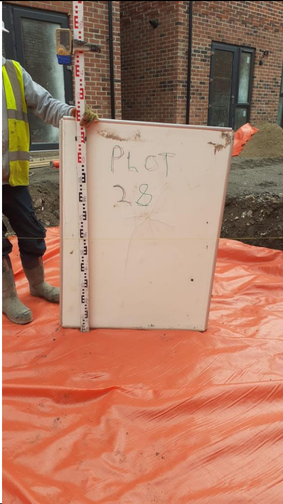
Photograph 12: Reduced level dig and membrane within rear garden of plot 28.
