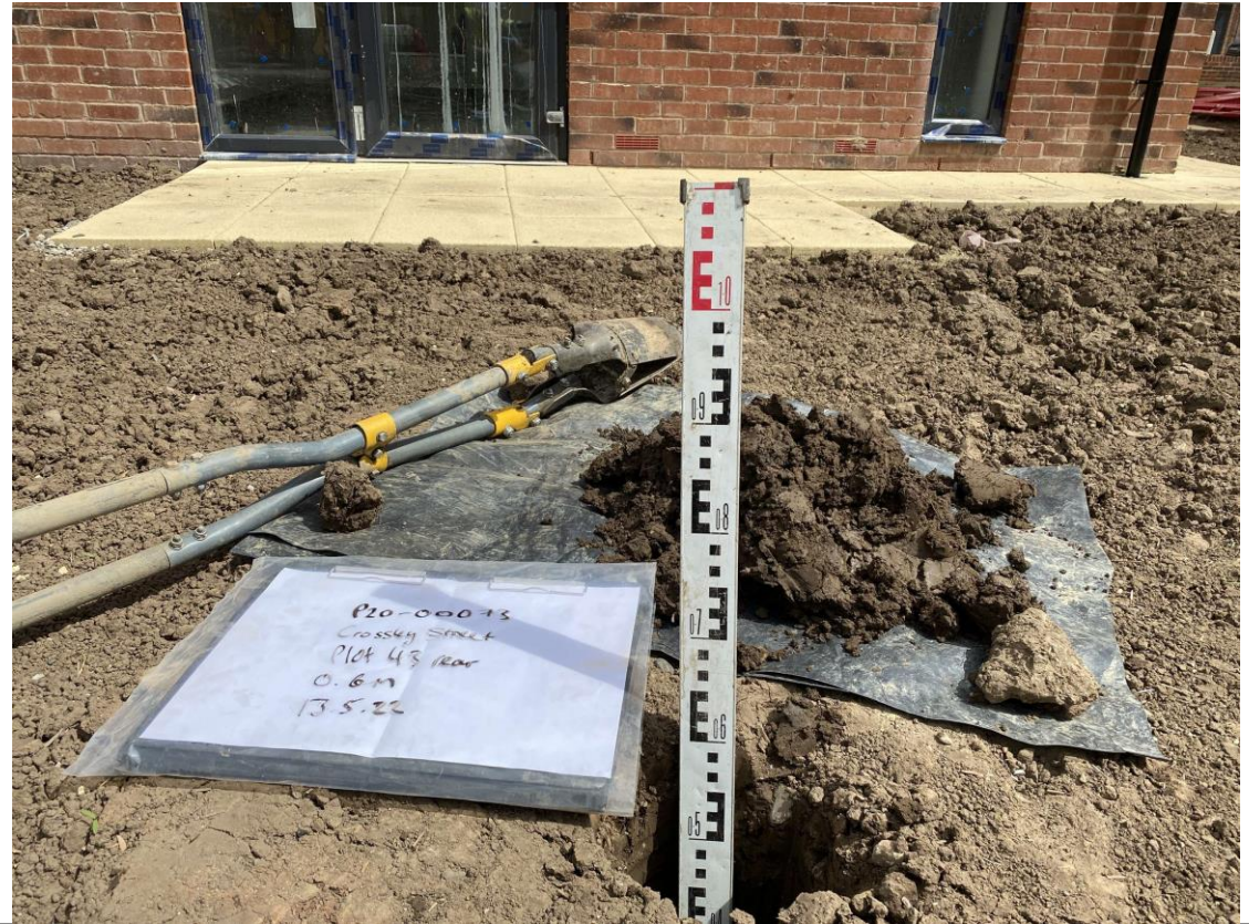
Photographs 3 and 4: Hand Dug Pit Topsoil Depth Validation – HDP16, Plot 43
