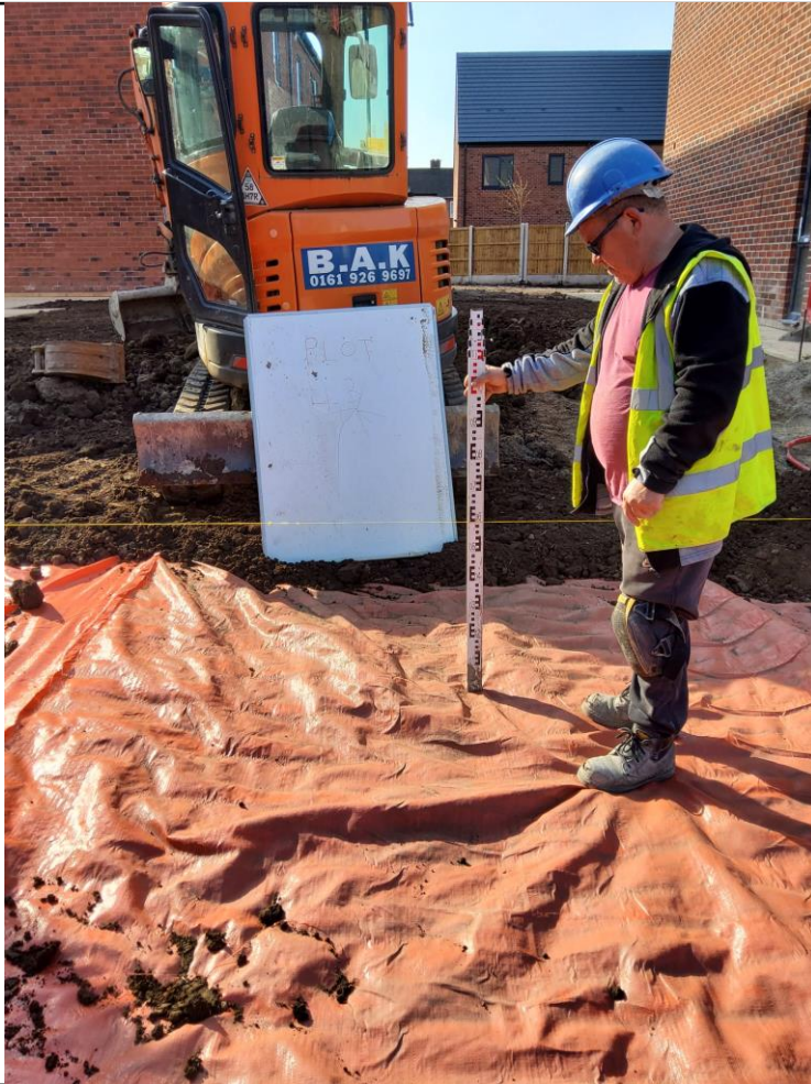
Photograph 16: Reduced level dig and membrane within rear garden of plot 43.
