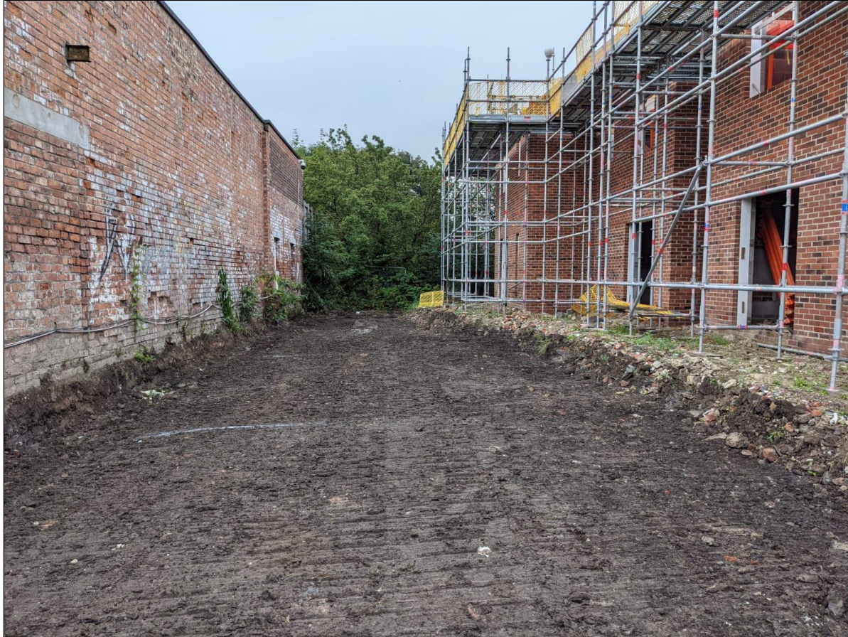
Photograph 1: Reduced level dig within rear gardens of plots 24-32.
