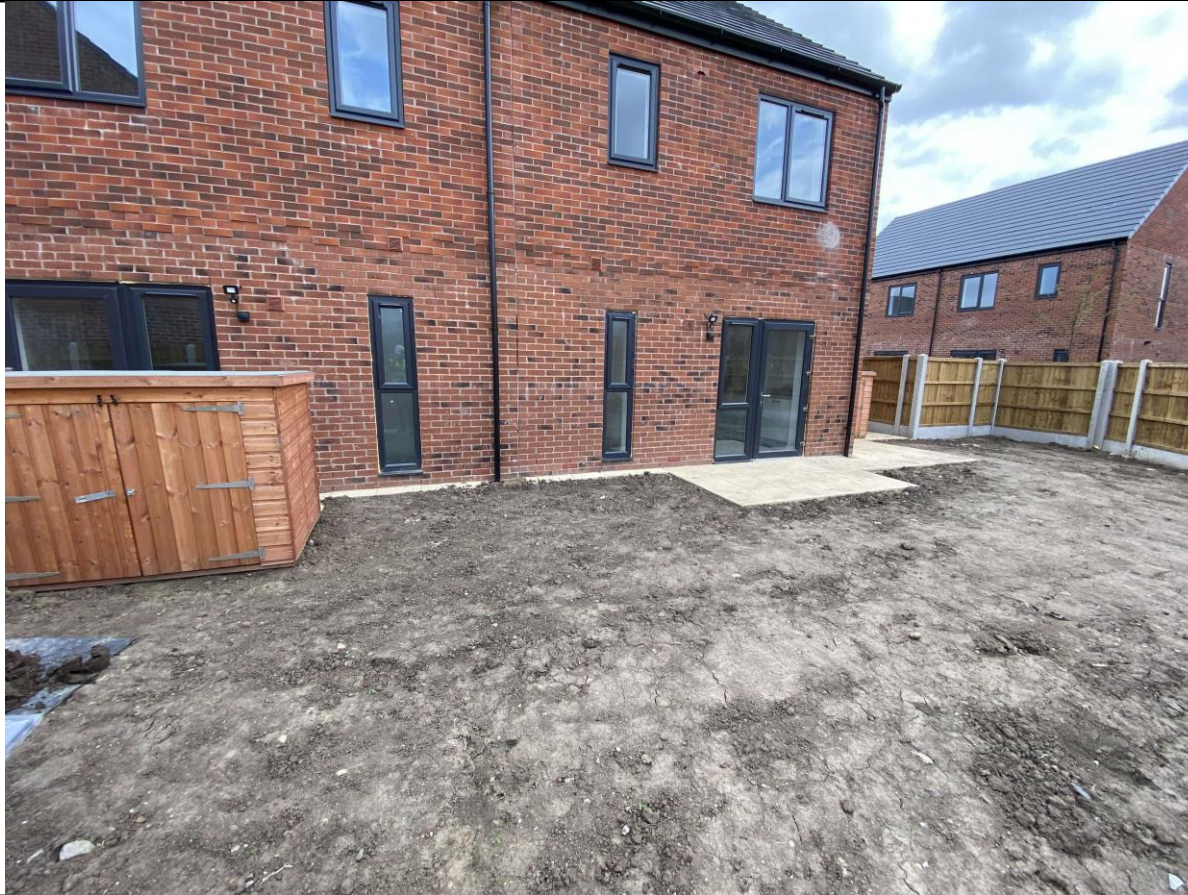
Photograph 8: Finished rear garden area of plot 45.
