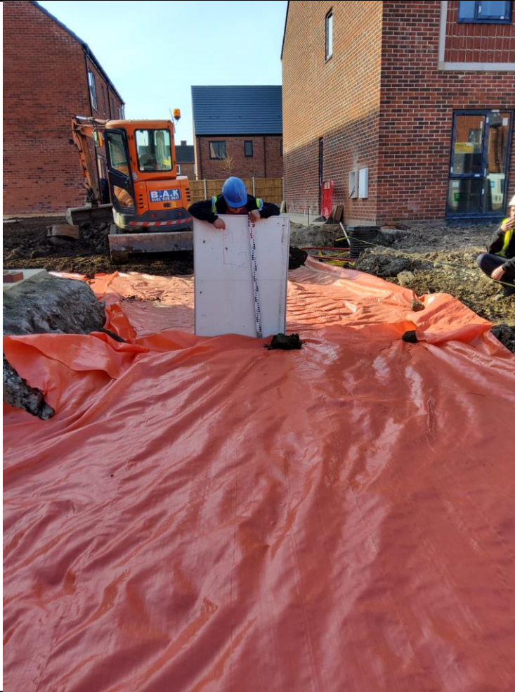
Photograph 14: Reduced level dig and membrane within rear garden of plot 42.
