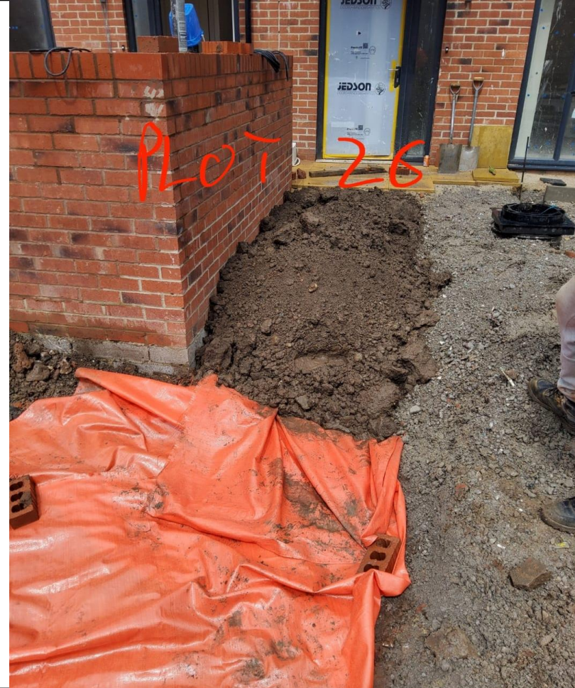
Photograph 10: Reduced level dig and membrane within front garden of plot 26.
