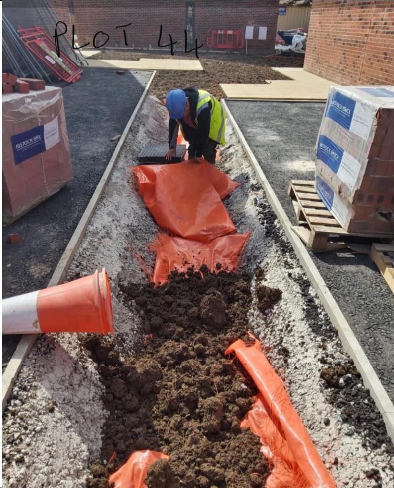
Photograph 20: Reduced level dig and membrane within front garden of plot 44.
