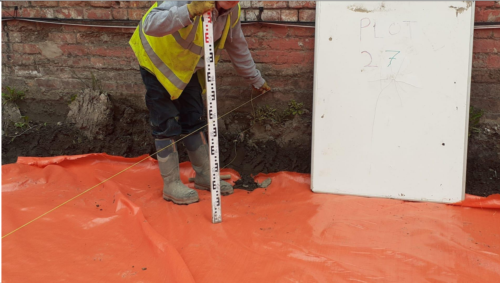
Photograph 11: Reduced level dig and membrane within rear garden of plot 27.
