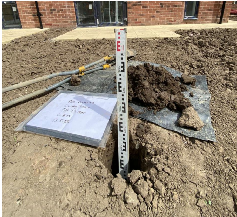
Photographs 3 and 4: Hand Dug Pit Topsoil Depth Validation – HDP16, Plot 43
