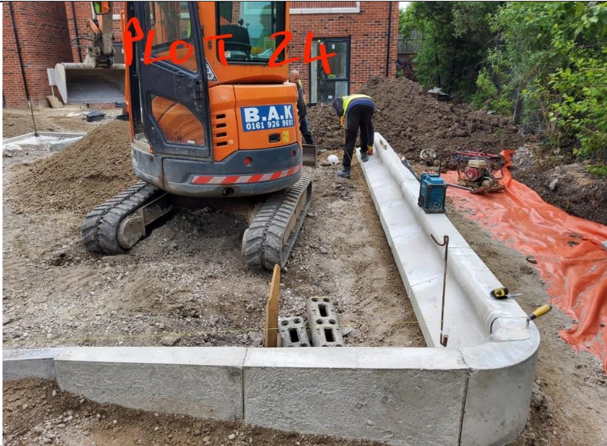
Photograph 5: Reduced level dig and membrane within front garden of plot 24.
