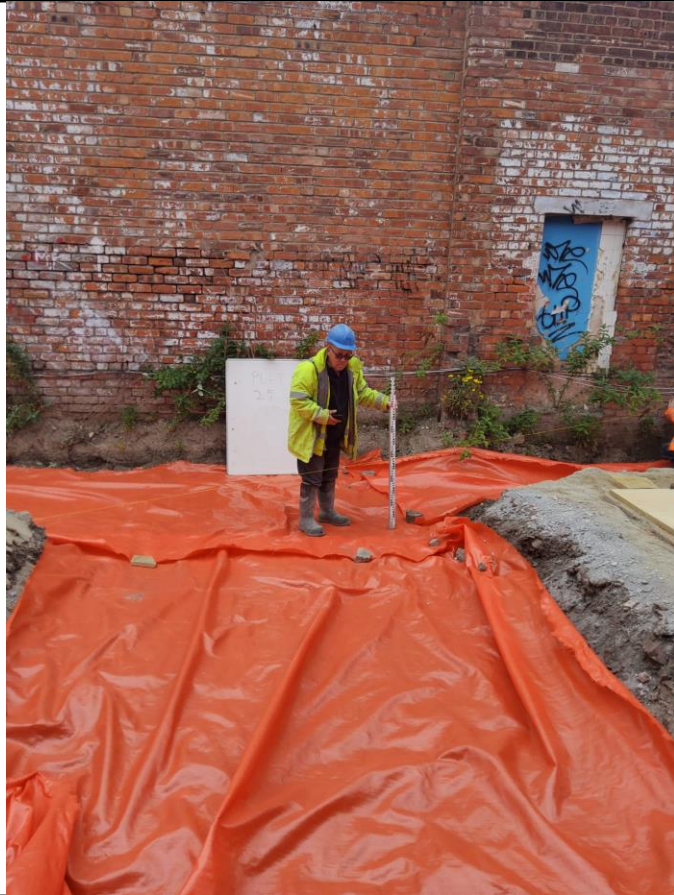
Photograph 7: Reduced level dig and membrane within rear garden of plot 25.
