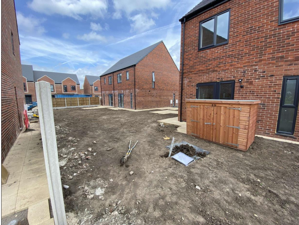
Photograph 8: Finished rear garden area of plot 44.
