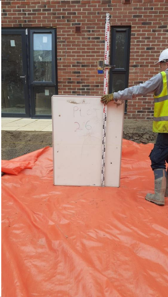
Photograph 9: Reduced level dig and membrane within rear garden of plot 26.
