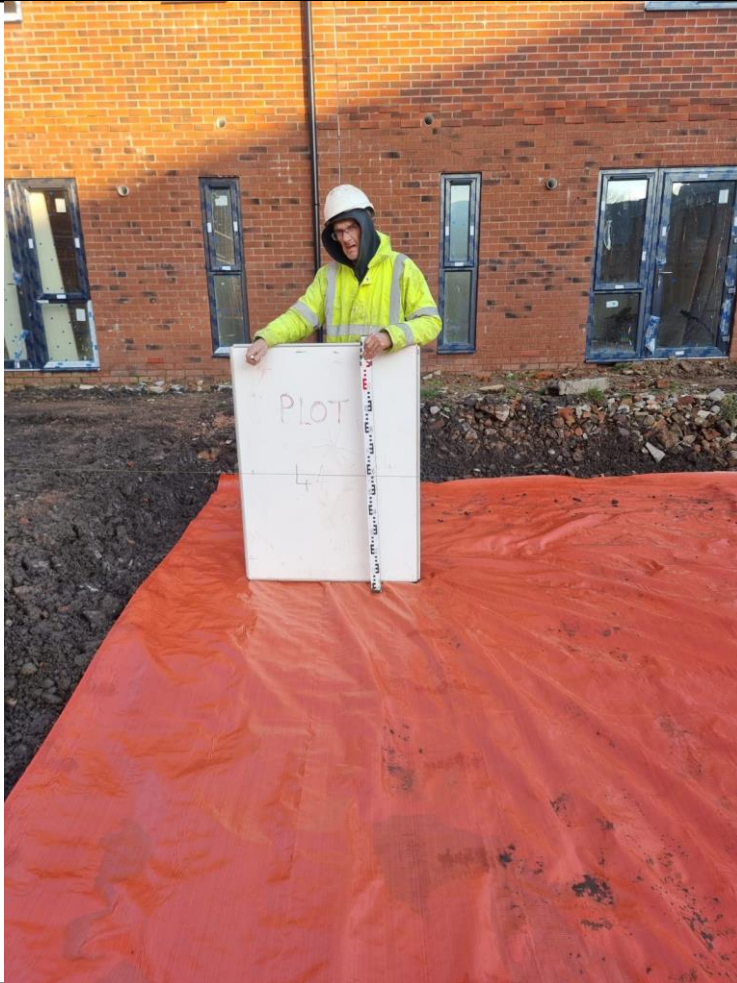
Photograph 18: Reduced level dig and membrane within rear garden of plot 44.
