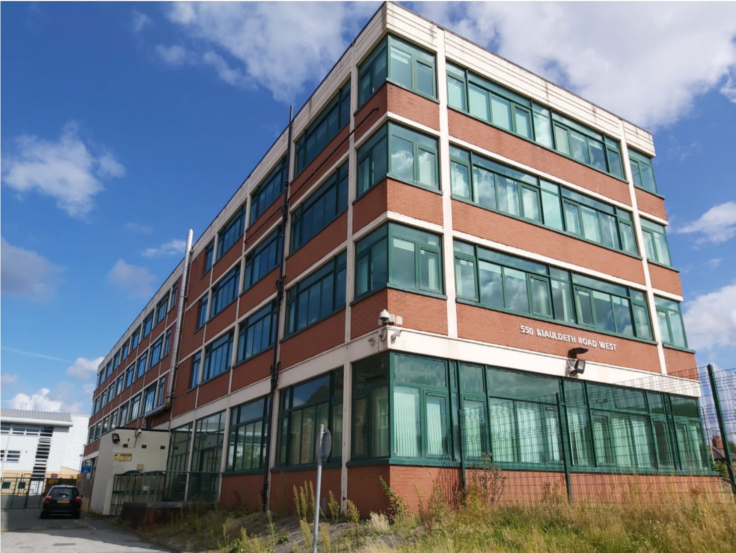
North West view of existing office block
