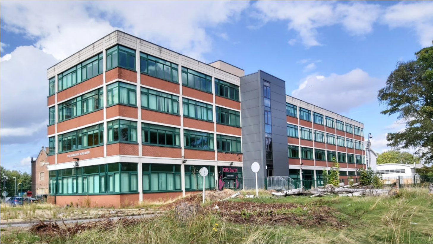
North East view of existing office block
