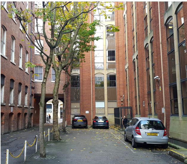
125 Portland Street Rear Parking Area
