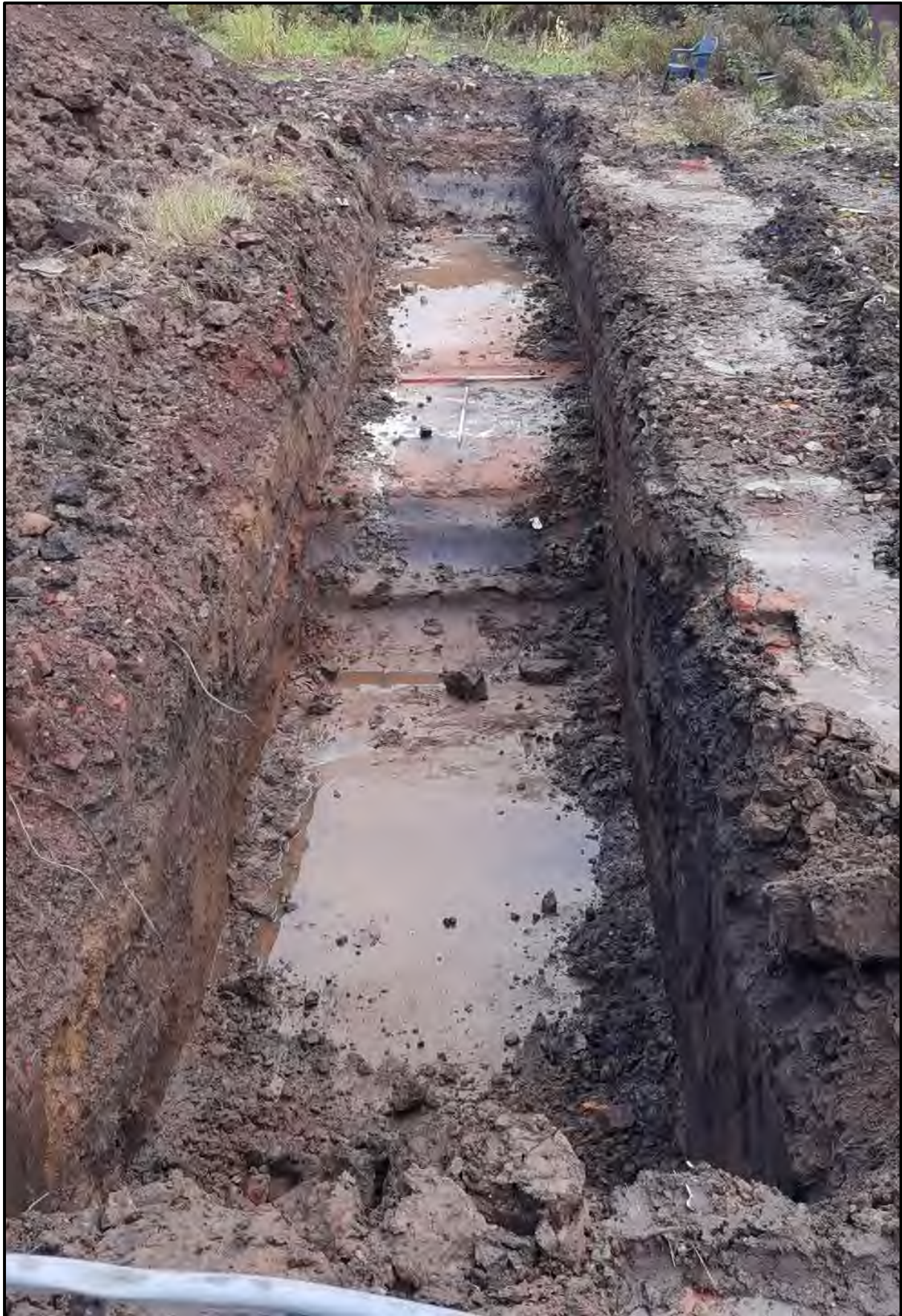
Plate Xx: A post-excavation view of Trench 11. Looking east.
