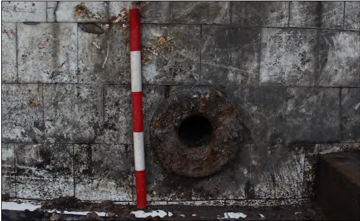
Plate xx: Cast iron collared pipe in pool 225 (0.50m scale)
