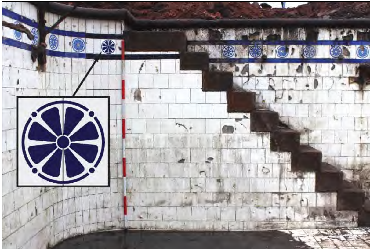
Plate xx: Pool 225 showing the later steps and replacement tiles (2m scale)
