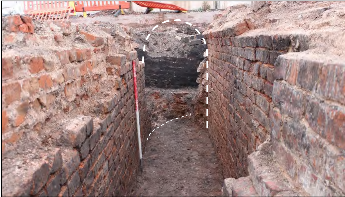
Plate _ View of the interior of the vaulted walkway 3069, looking north (1m scale). Note the remains of the curved outer wall preserved beneath a later raised floor surface within flue 3064 to the north, and the surviving vaulting that was an original feature of both 3069 and 3064
