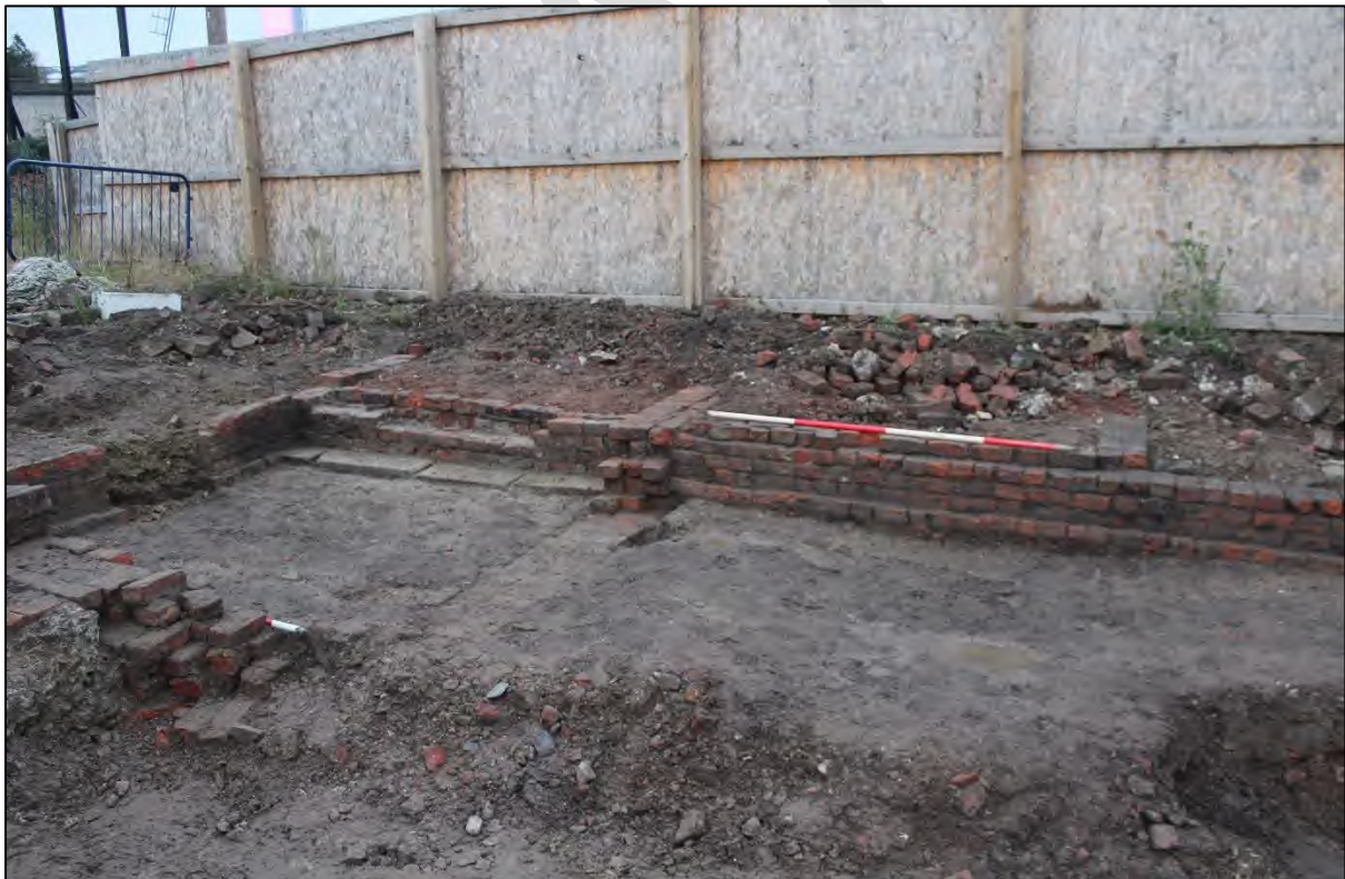
Plate xx: Wall 223 looking west (2m scale)
