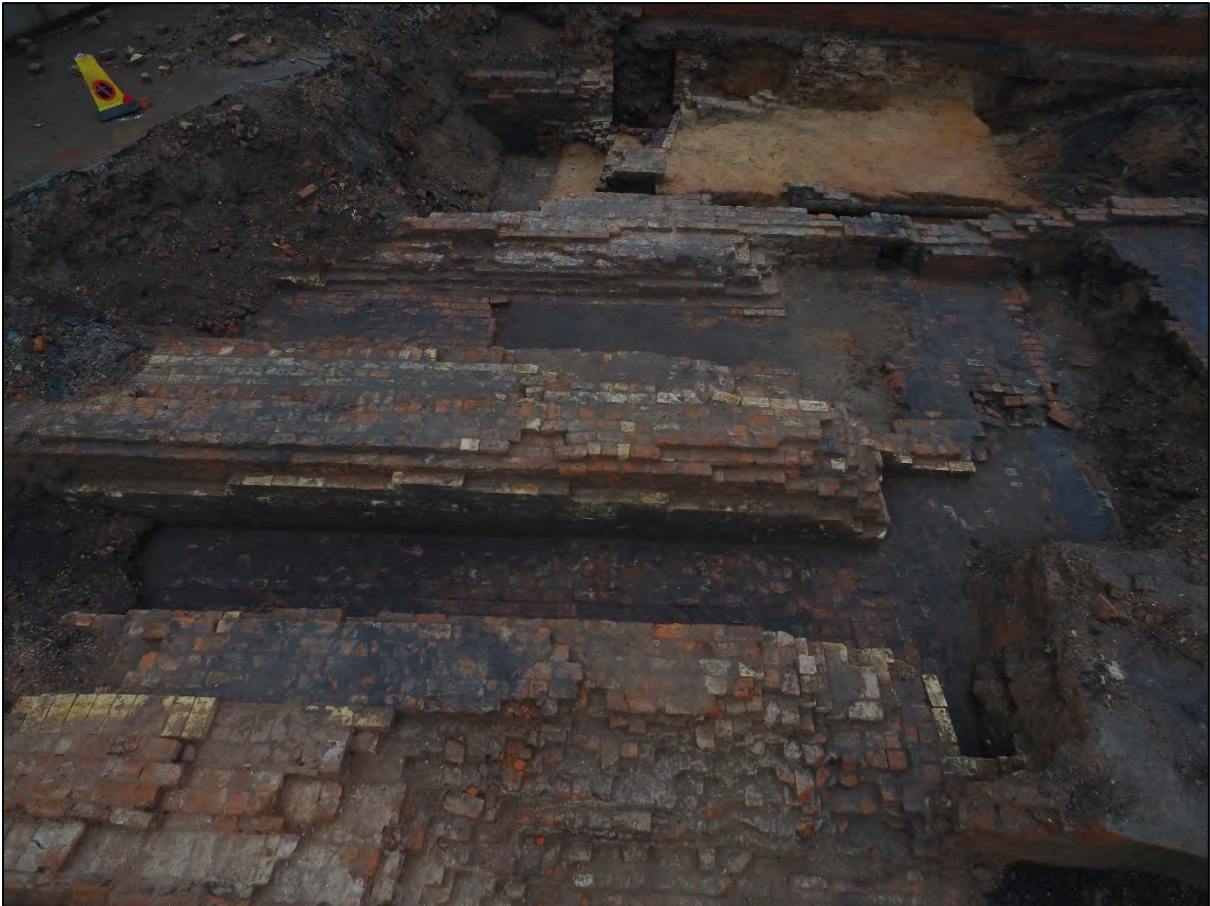
Plate_ Aerial view across boiler beds 3061 and 3060, looking east towards the economising house
