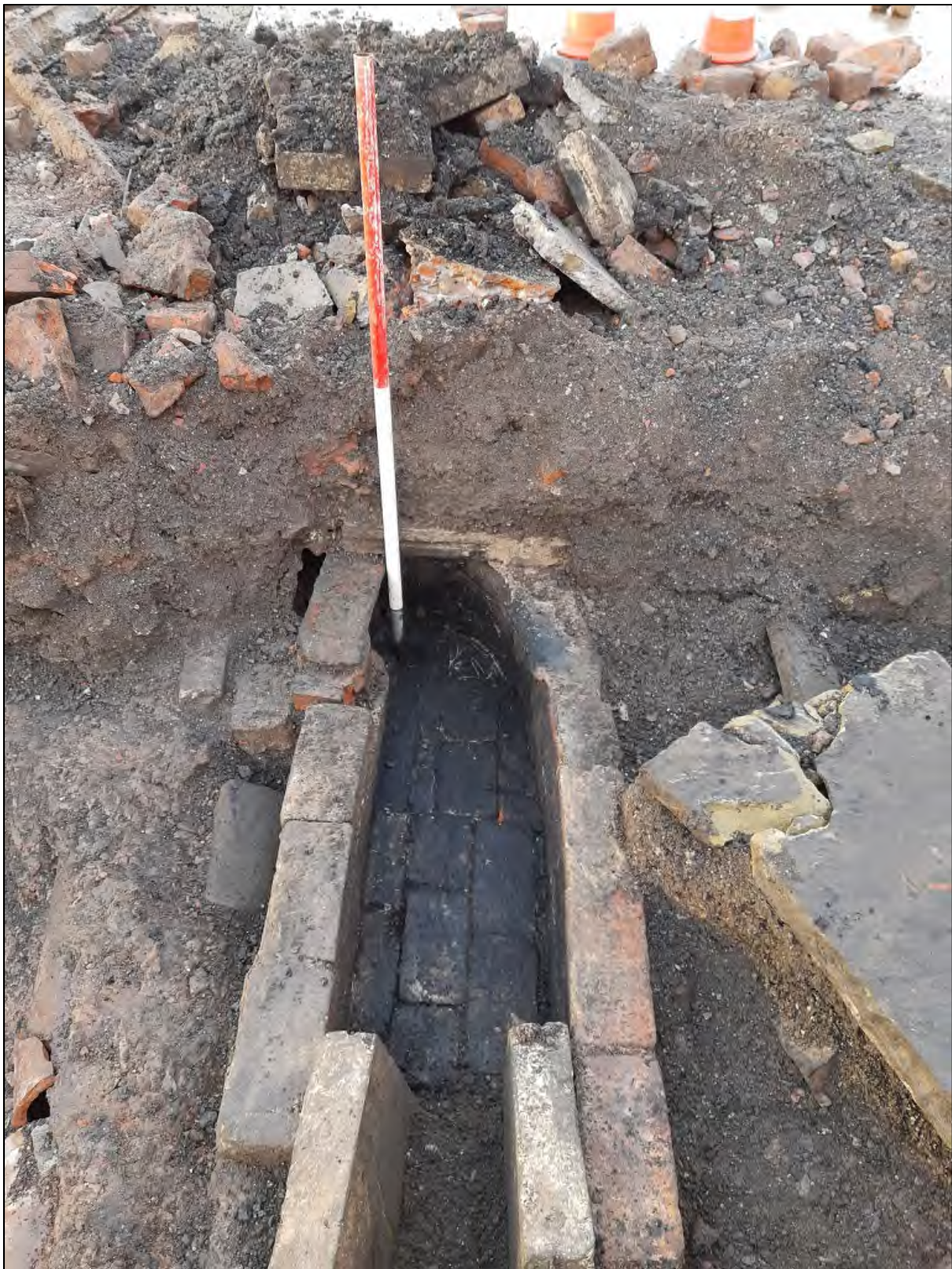
Plate xx: Structure 0202. Note the brick base to the flue and the sharp eastwards curve into the southern limit of the excavation.
