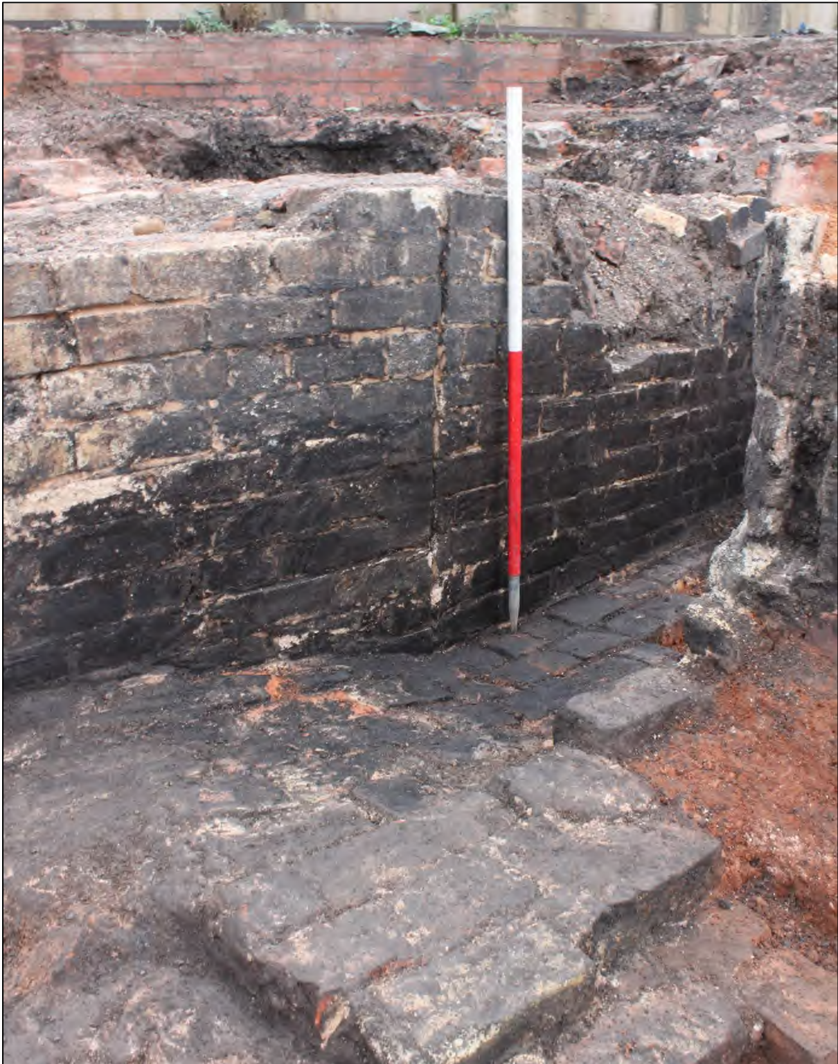
Plate_ : Vertical phase break within the northern wall of flue 3064 indicating its point of extension (1m scale). Note the upward sloping floor within the flue.
