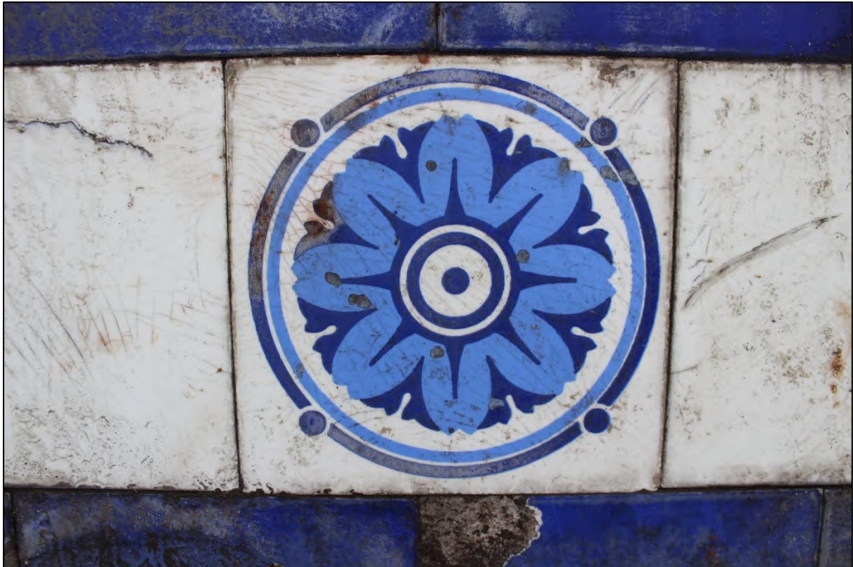
Plate xx: Example of the Minton Hollins and Co. tile used in the retiling of pool 225
