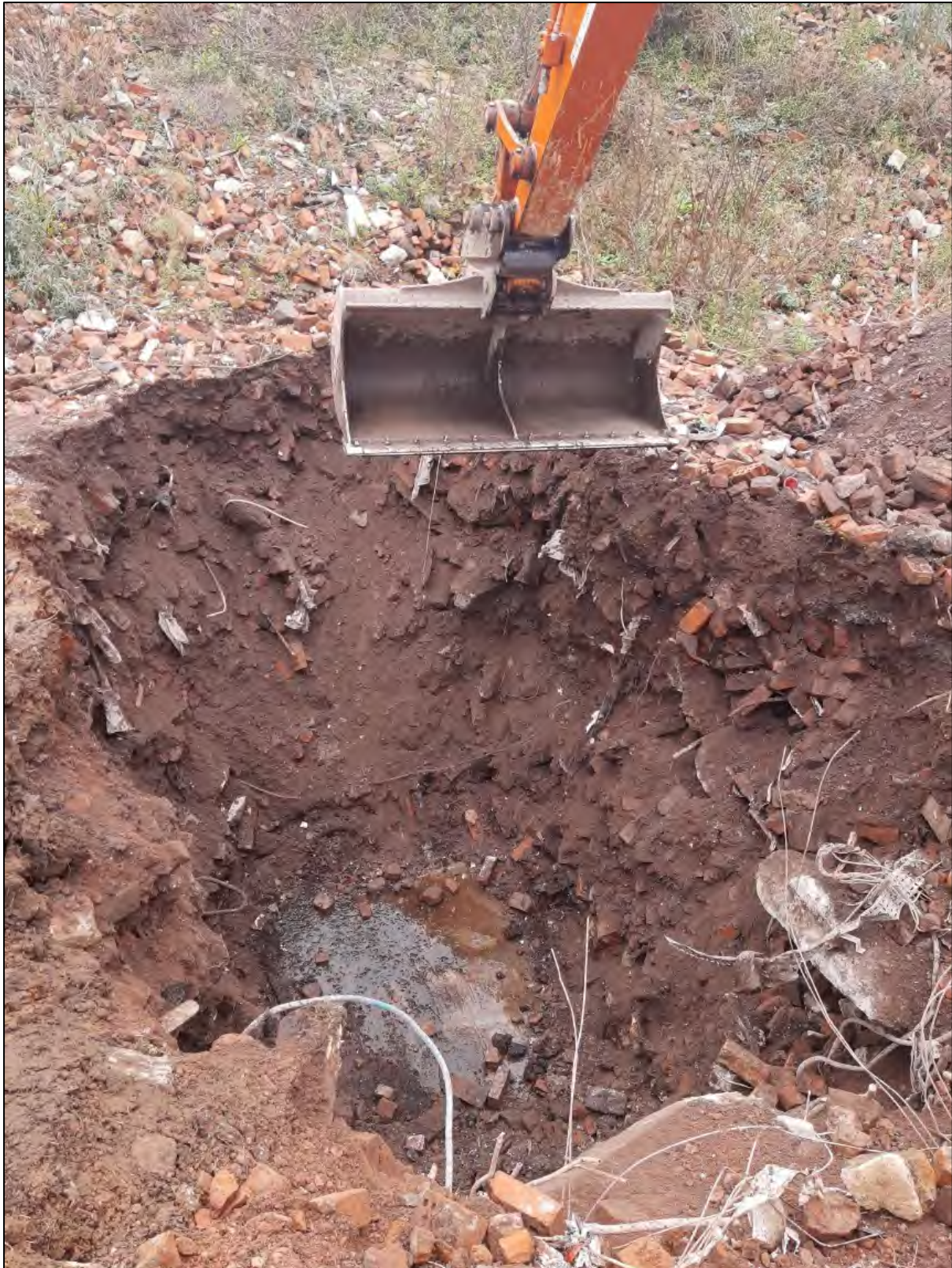
Plate xX: A mid-excavation shot of Trench 9, illustrating that the entirety of the trench had been heavily remediated. Looking south.
