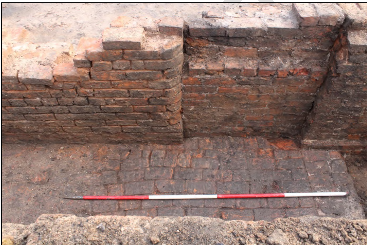
Plate_ : Southern end of the excavated walkway 3069, showing the blocked doorway 3177 (2m scale)
