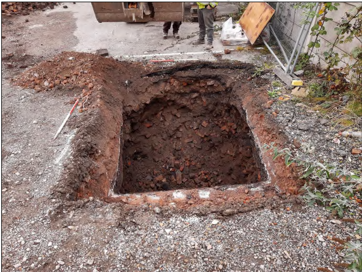
Plate xx: A post-excavation shot of Trench 1, illustrating the level of remediation that was uncovered. Looking southeast.
