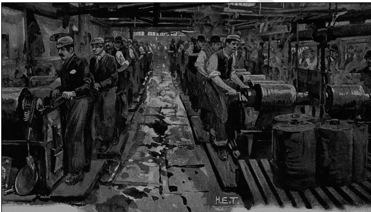
Plate x: Dye house in Messrs Worrall's works, Manchester
