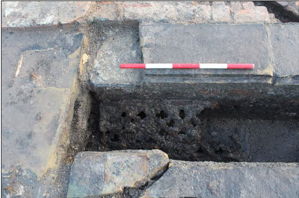
Plate_ : Detail of drain interior, rebated stone coping and collapsed cast-iron grate
