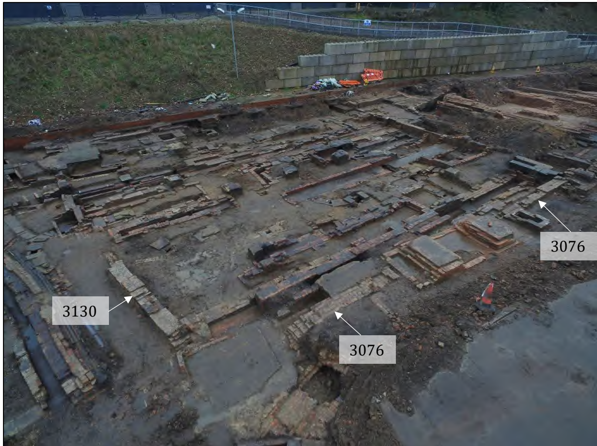
Plate__: View across the southern half of Building C indicating the Phase 3 walls 3130 and 3076
