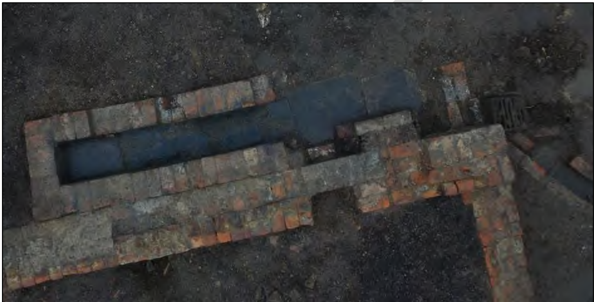
Plate __: Sub-aerial view of slate-lined drain 3039 with part of drain 3052 visible to the east, looking north
