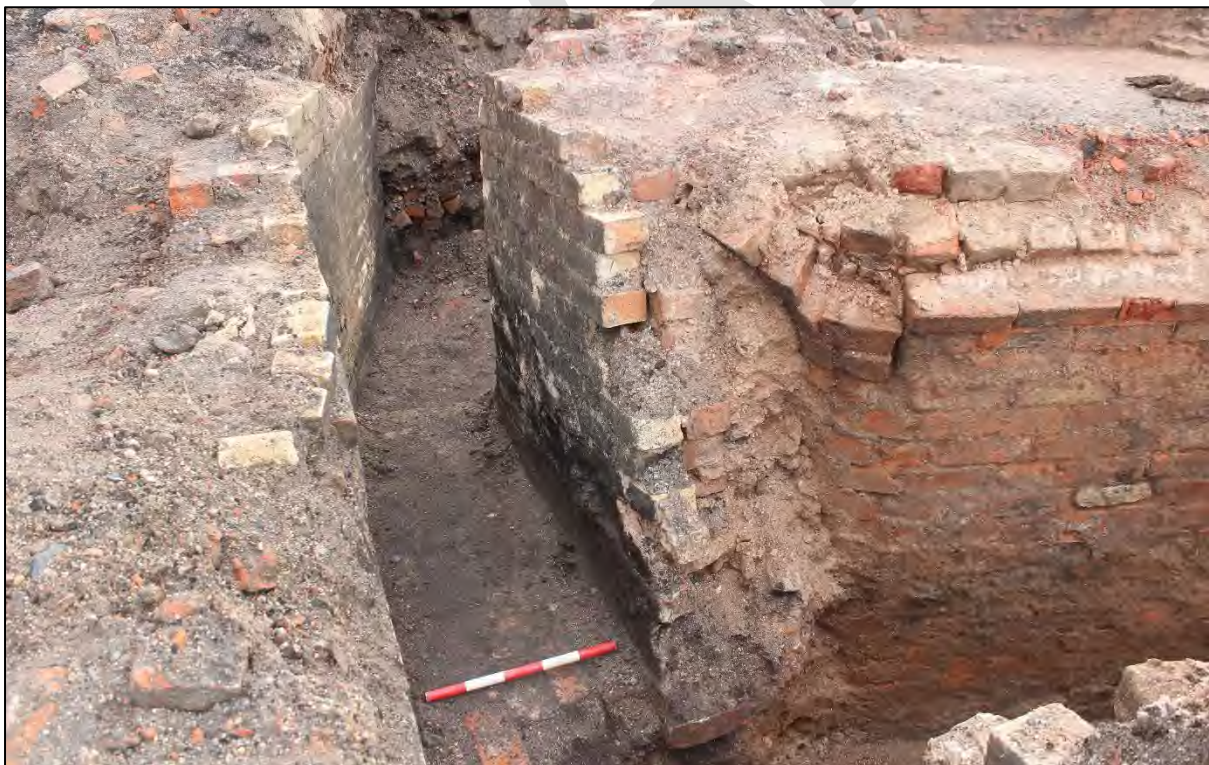
Plate_: View of Flue 3064 and walkway 3069, looking east (0.50m scale)
