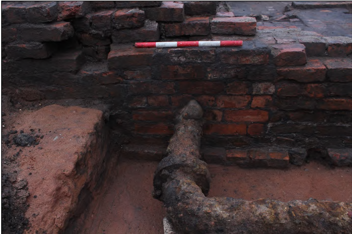
Plate_: The cast iron pipe and Phase 5 repair to the southern extent of wall 3070, note the use of a black mortar
