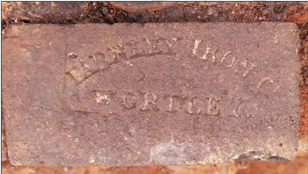
Plate xx: Firebrick bearing the stamp Farnley Iron Co. Wortley' utilised in Boiler 111
