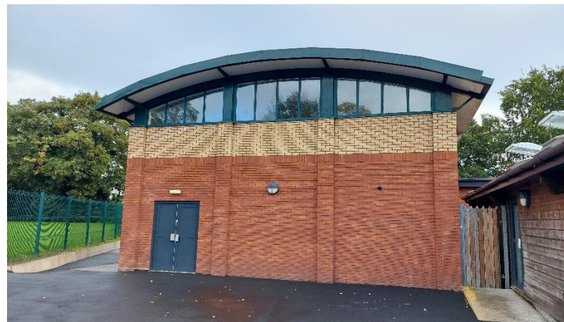
Photograph 6: Large gym building at SJ 81598 90676. Negligible suitability.
