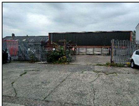
Plate 2: View, facing south into the Site access gate
