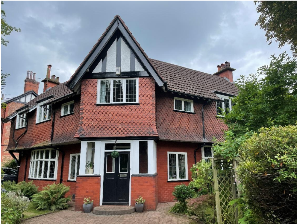
View from Parkfield Road South Road/Oriel Road corner (Looking south west)
