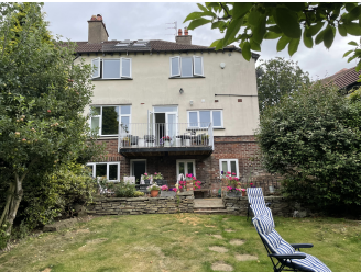
Photograph of existing rear facade
