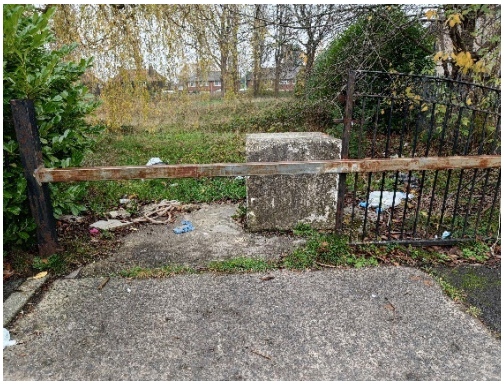
Photograph 1: Steel gate, southeast of the site, providing vehicular access to the development.
