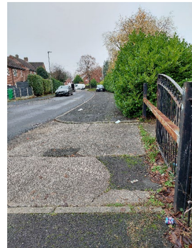
Photograph 6: Street lighting present on Benmore Road and view west of the site.
