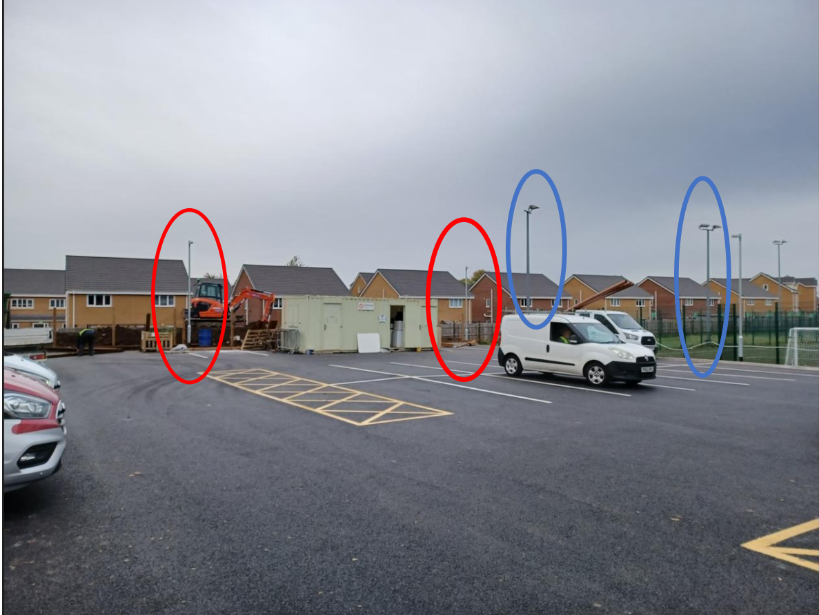
View northwards across car park, lighting columns proposed circled red, existing taller columns in blue
