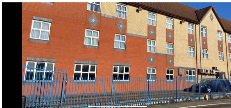
Existing façade onto Kirkmanshulme Lane
