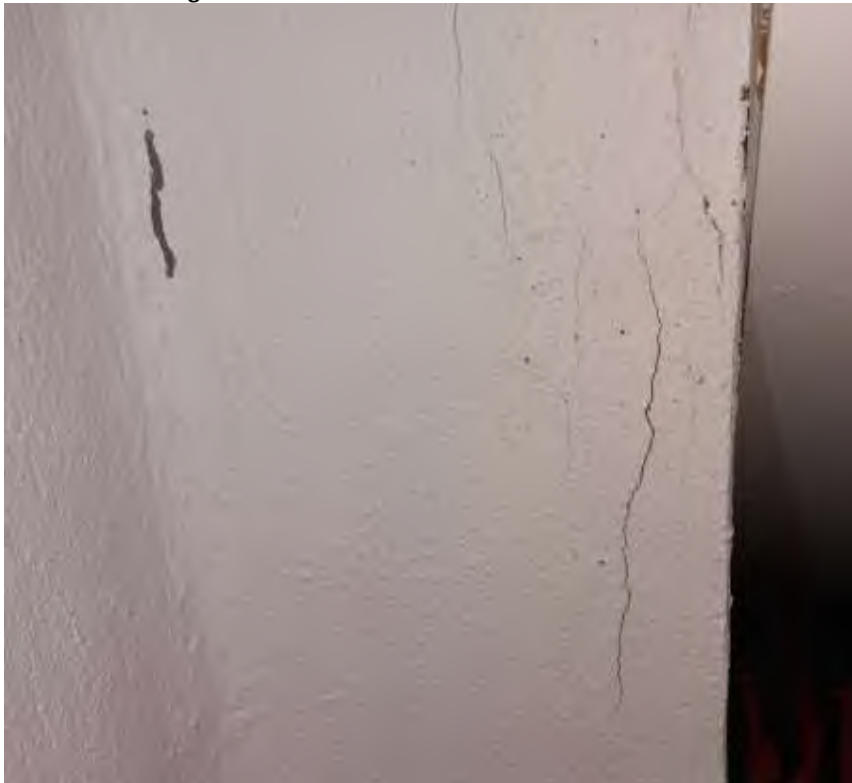
Render cracking local to corner bead:
