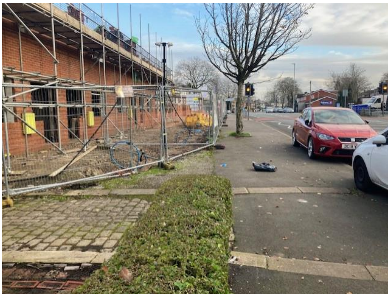
View of the site area enclosed by Heras fencing
