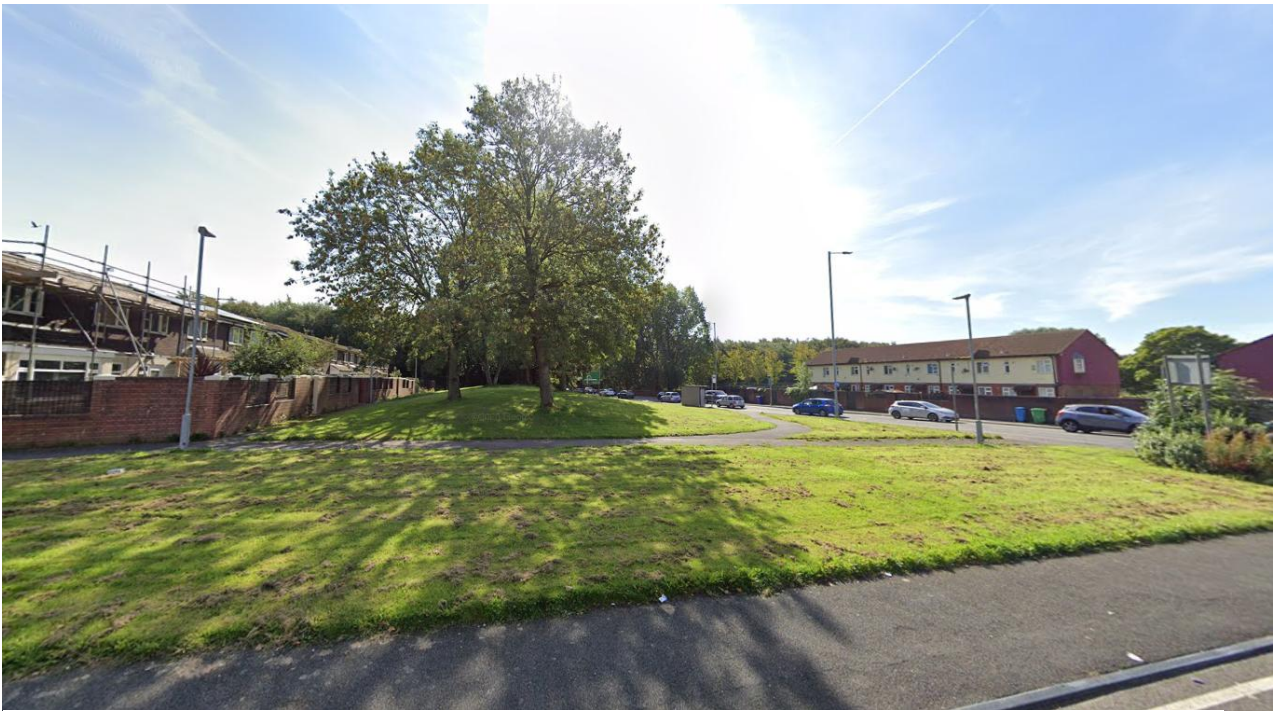
View of Site from Sedgeford Road
