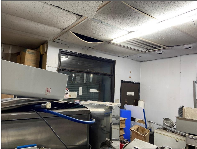
Photograph 20 showing the office space at the rear of the building
