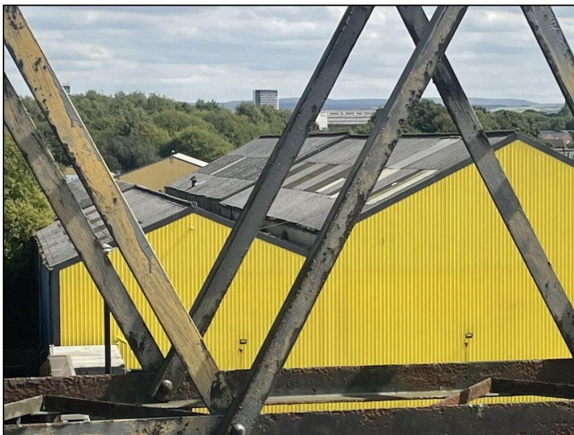
Photograph 7 showing the roof of units 1 and 2
