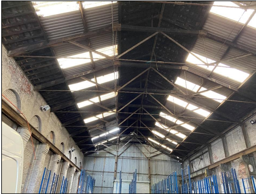
Photograph 14 showing the interior space of Unit 3
