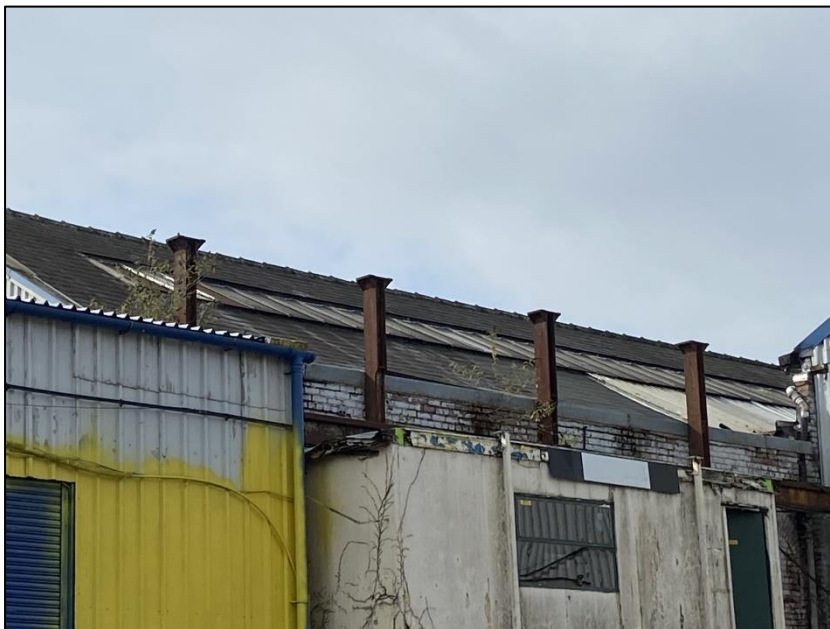
Photograph 18 showing the roof of Unit 4
