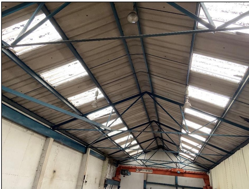
Photograph 12 showing the roof void above the main house
