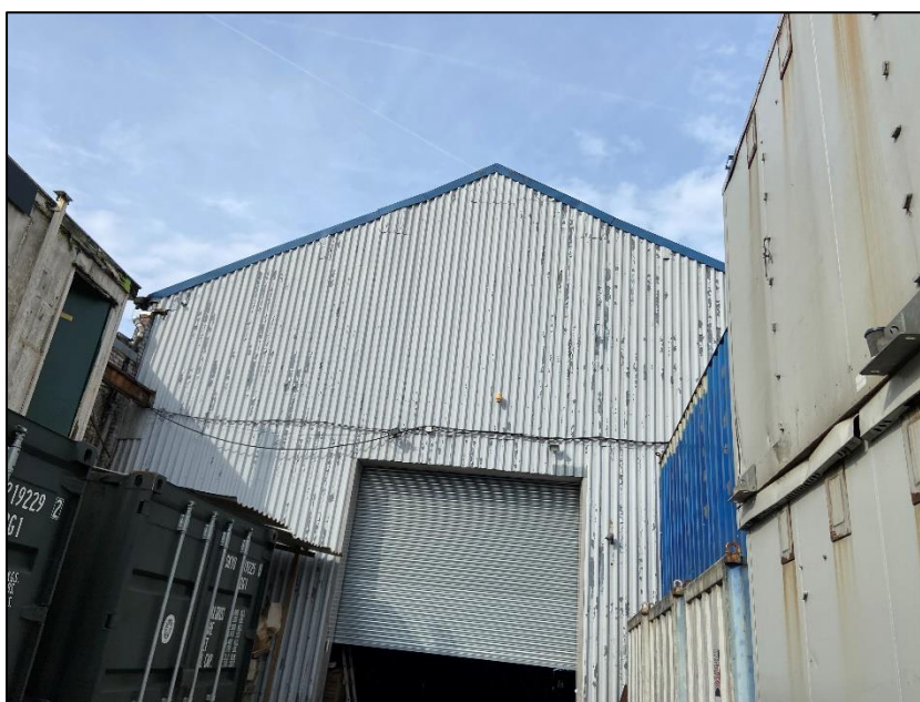
Photograph 14 showing eastern gable end of Unit 3
