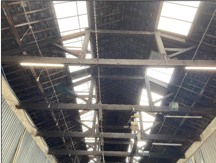
Photograph 19 showing the internal space of Unit 4
