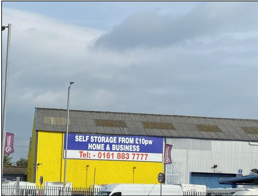
Photograph 8 showing the roof of unit 2
