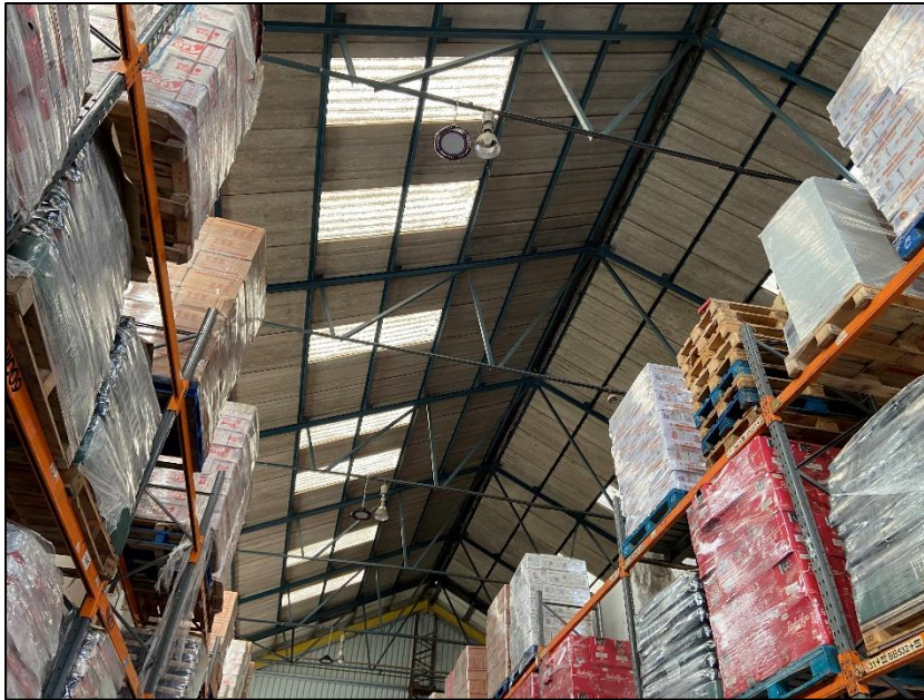
Photograph 11 showing the internal space of Unit 7
