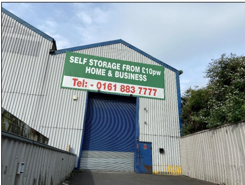
Photograph 5 showing metal cladding and one of the access doors
