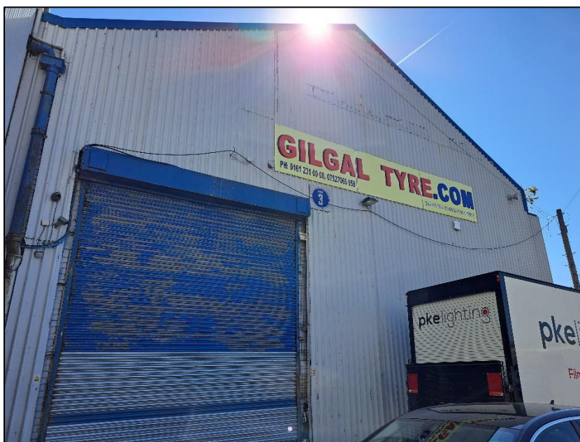
Photograph 13 showing the western gable end of Unit 3
