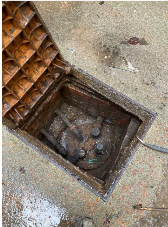
PLATE 7 TANK SERVICE MANHOLE – CENTRAL COURTYARD
