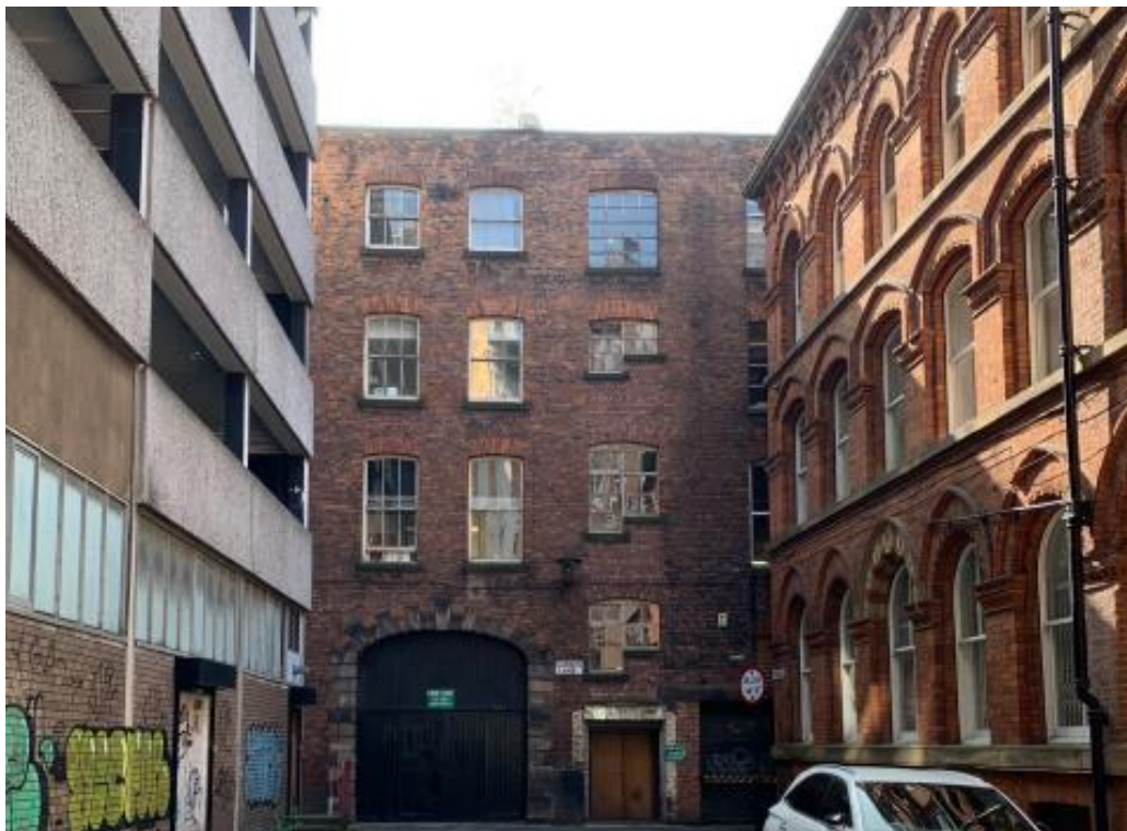
PLATE 3 VIEW OF BUILDING AND GATE IN THE NORTH FROM GARDEN LANE
