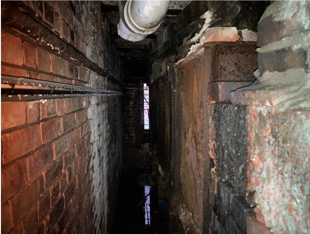
PLATE 5 UNDERGROUND STORAGE TANK
