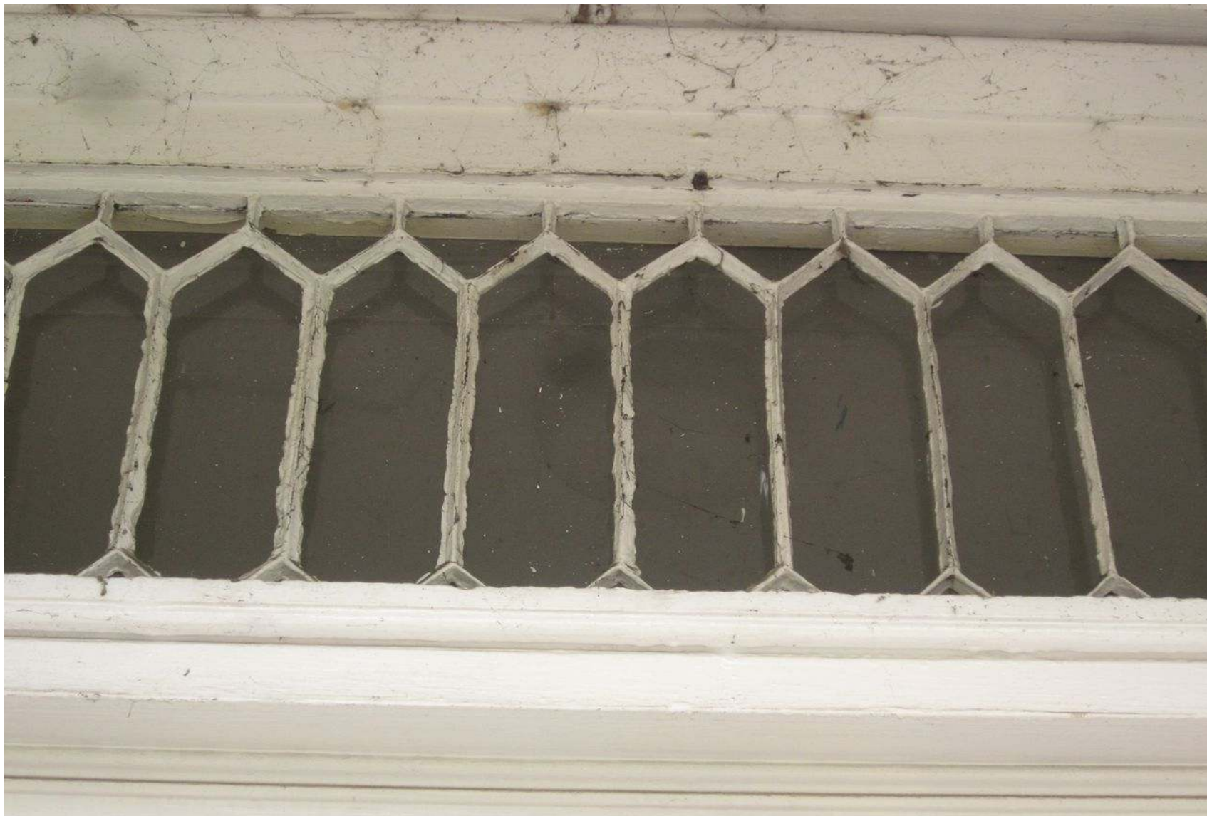
Original Vestibule Fanlight Glazing
