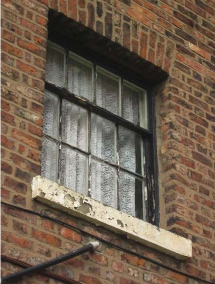
Original existing 12-pane top sash window
