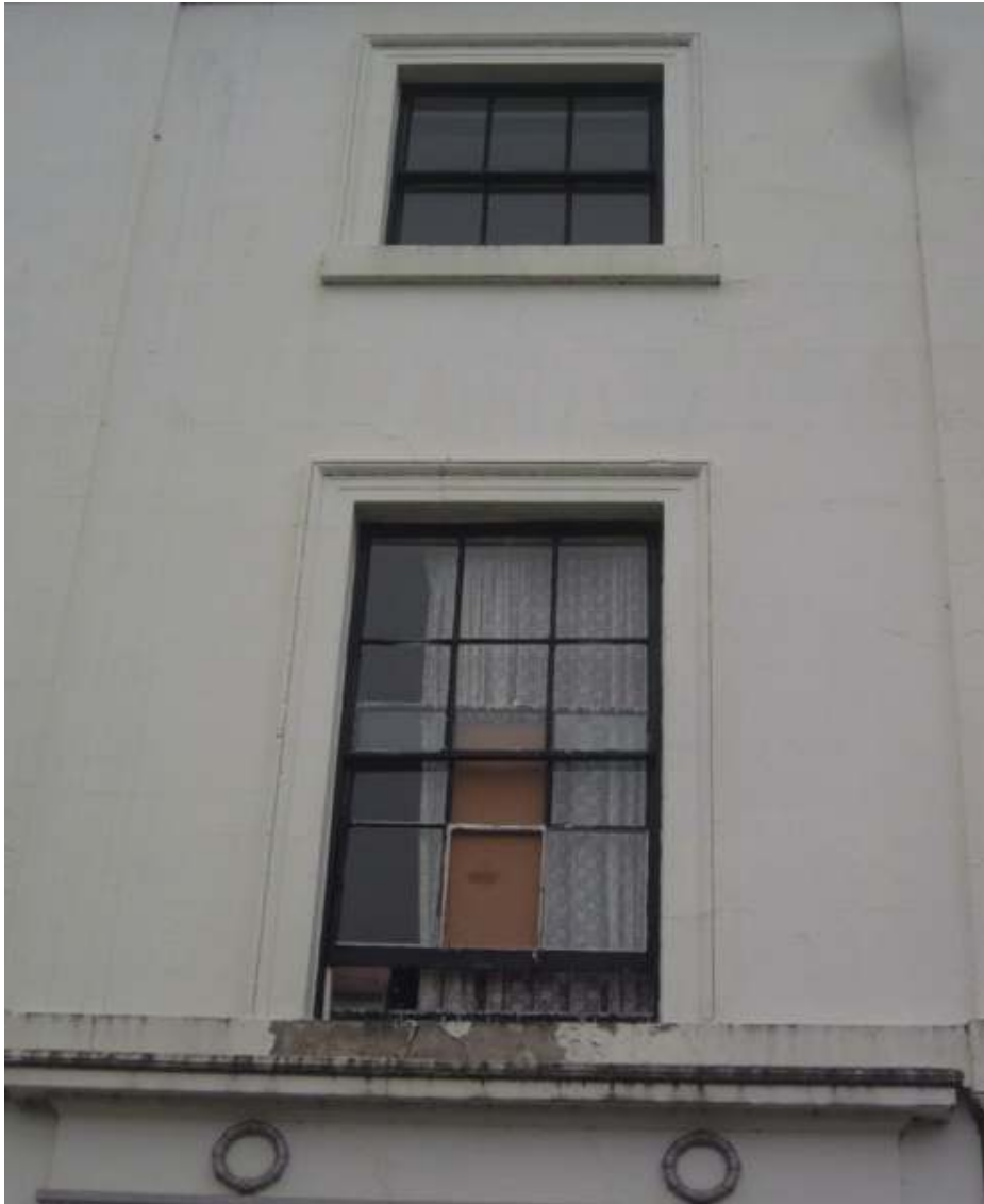
Original Timber Sash Windows to front elevation
