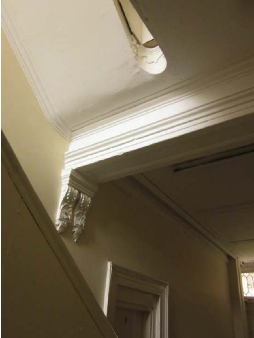
Plaster Cornices & Timber skirting board
