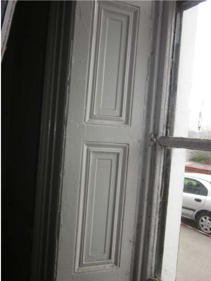
Timber Panneling – Window Shutters
