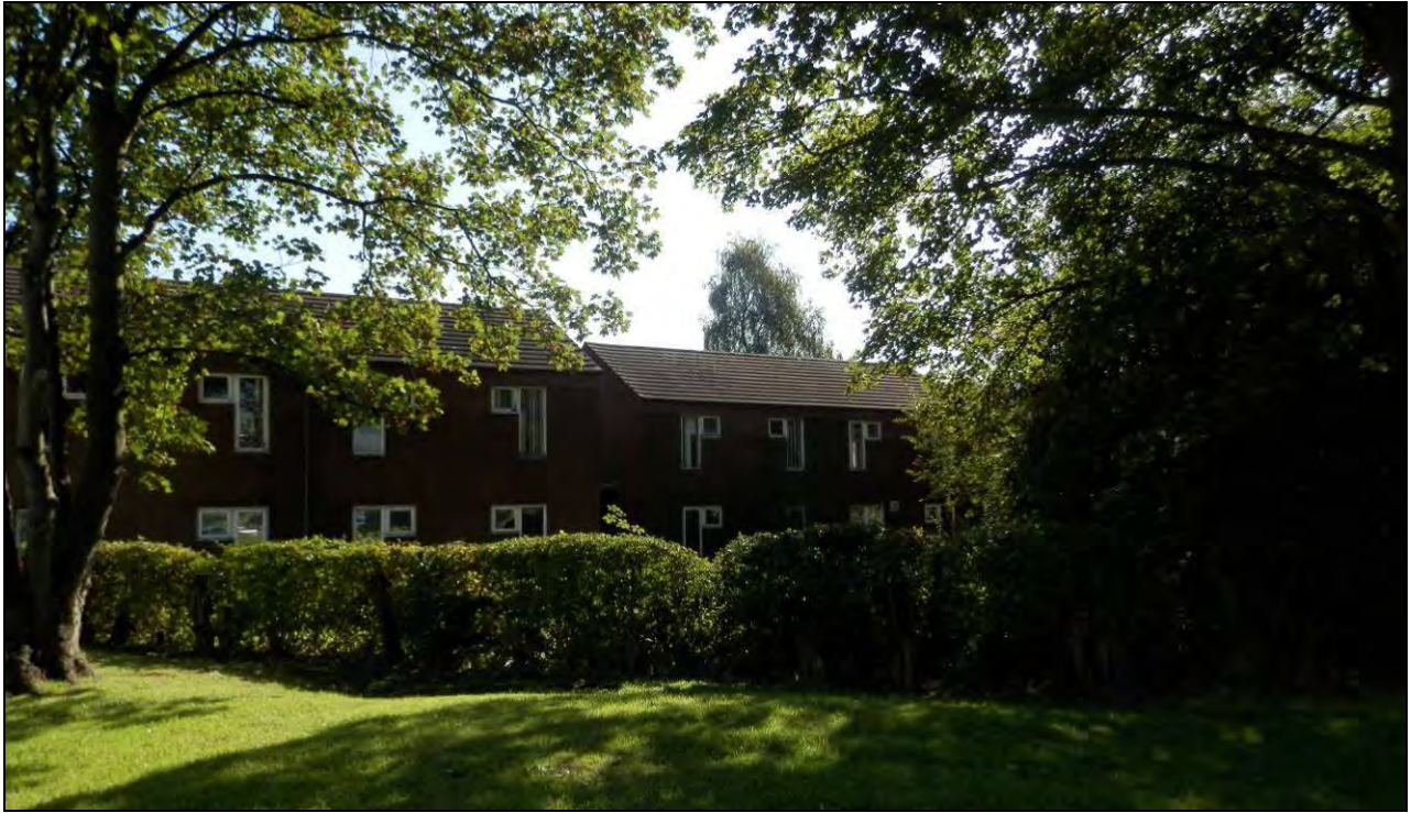
Photograph 5: Former residential building to the northeast of the site
