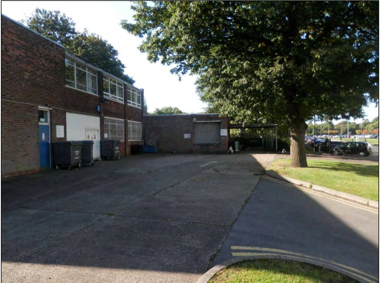
Photograph 4: Older technical building to the northeast of the site
