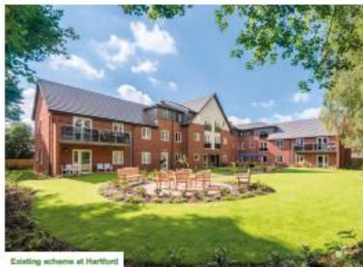
Existing scheme at Hartford
