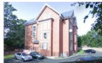
Four storey corner turned with full height gable on side with three storey square bay.
