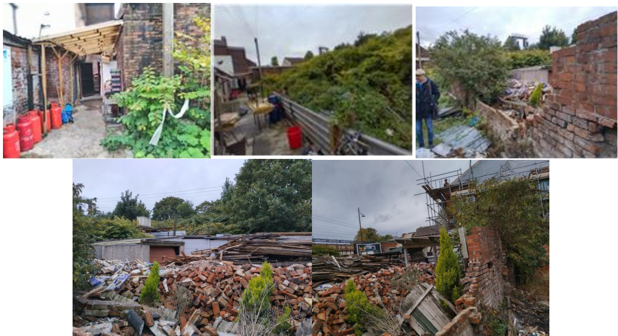
Fig.2 – Views of the application site (Building 1)
