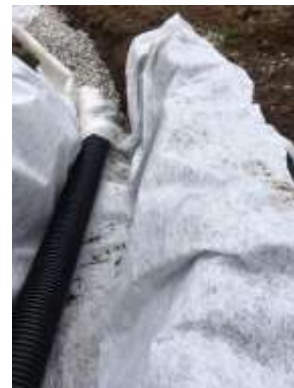
Photo 4: French Drain installation.
