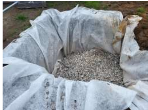
Photo 2: Soakaway installation.
