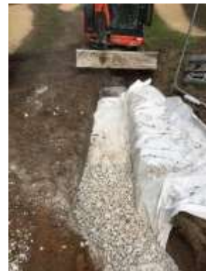
Photo 6: French Drain installation.
