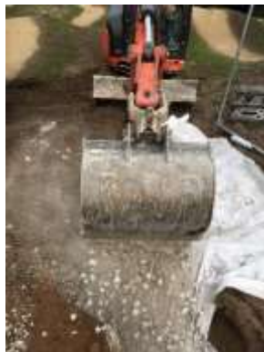
Photo 5: French Drain installation.
