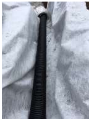
Photo 3: French Drain installation.
