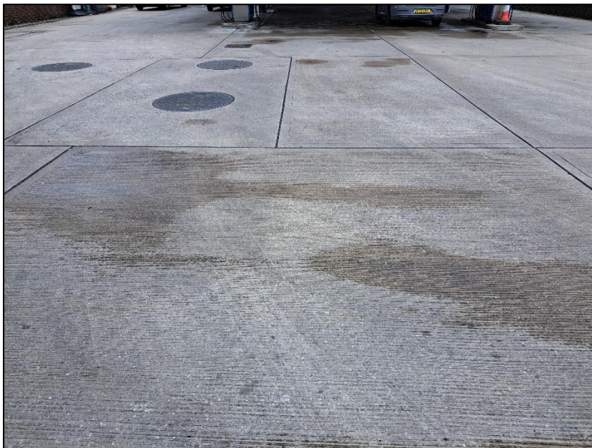
Photograph 7 showing the bare ground
