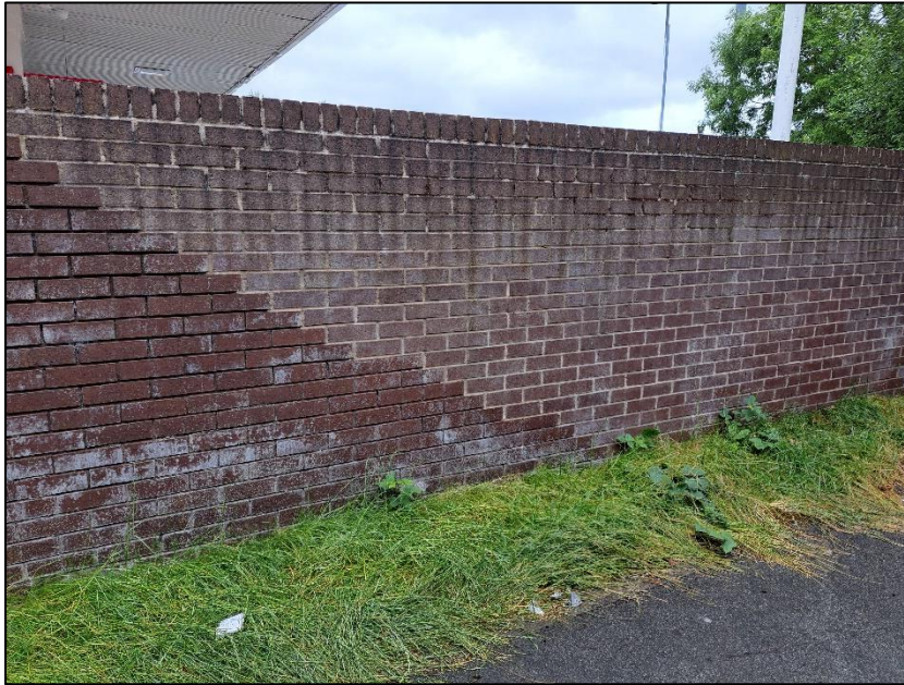
Photograph 8 showing the walls
