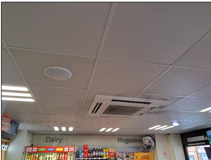
Photograph 14 showing the ceiling tiles
