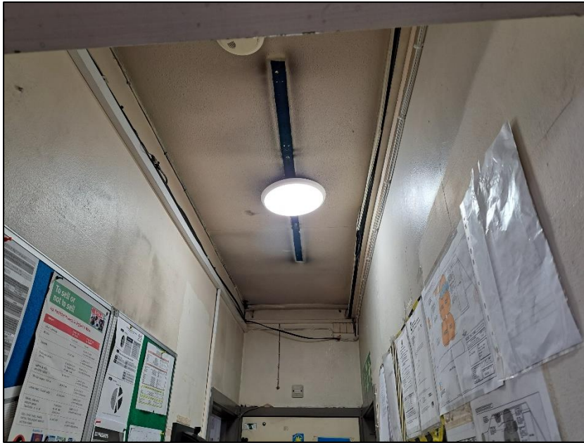
Photograph 13 showing the ceiling of the building from the interior
