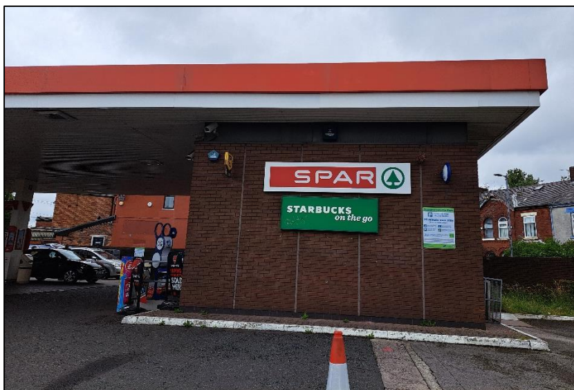
Photograph 11 showing the retail unit brickwork
