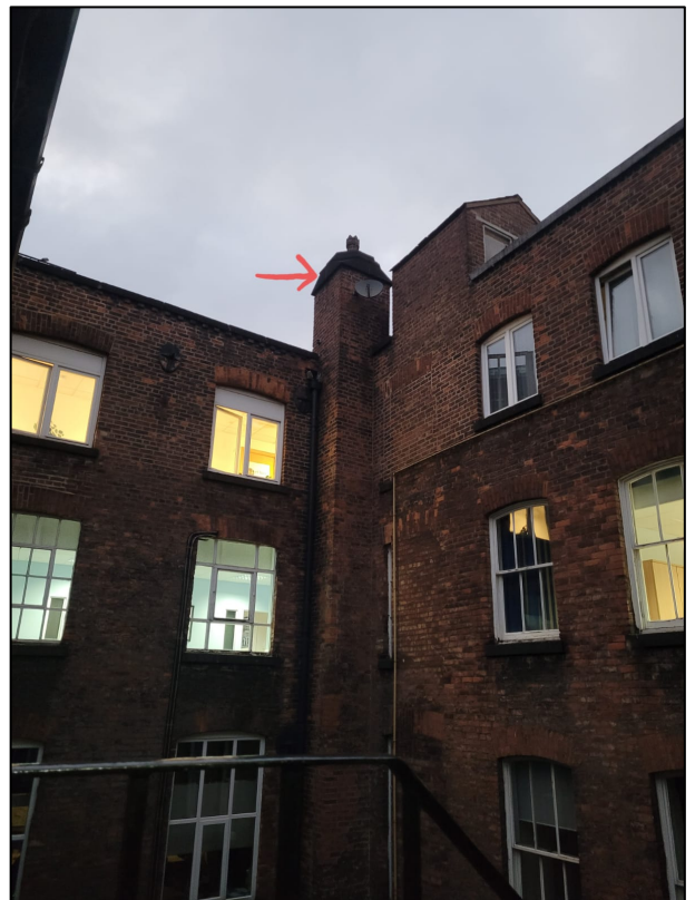
Photo 9 Location of confirmed Roost in courtyard chimney
