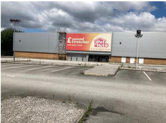
View of the front of the building when viewed from the front car park
