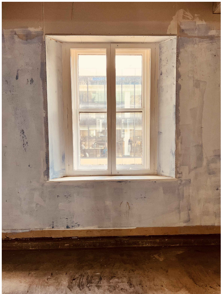
01 THIRD FLOOR EXISTING SECONDARY GLAZING TO BE UPGRADED 575 SCALE - N/A PHOTOGRAPH
