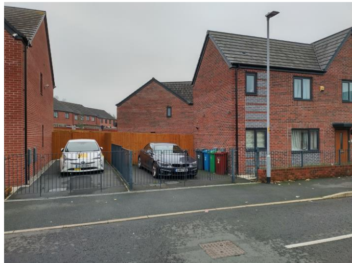
Fig.2 – Front elevation and boundary with 4 Lilford Close
