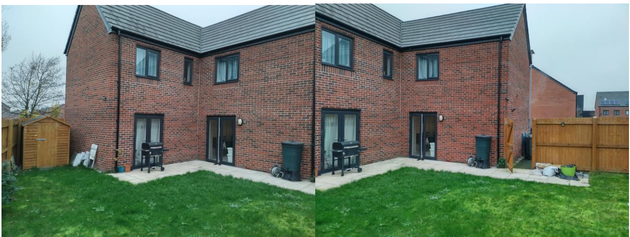
Fig. 3 – Rear elevation 2 Lilford Close
