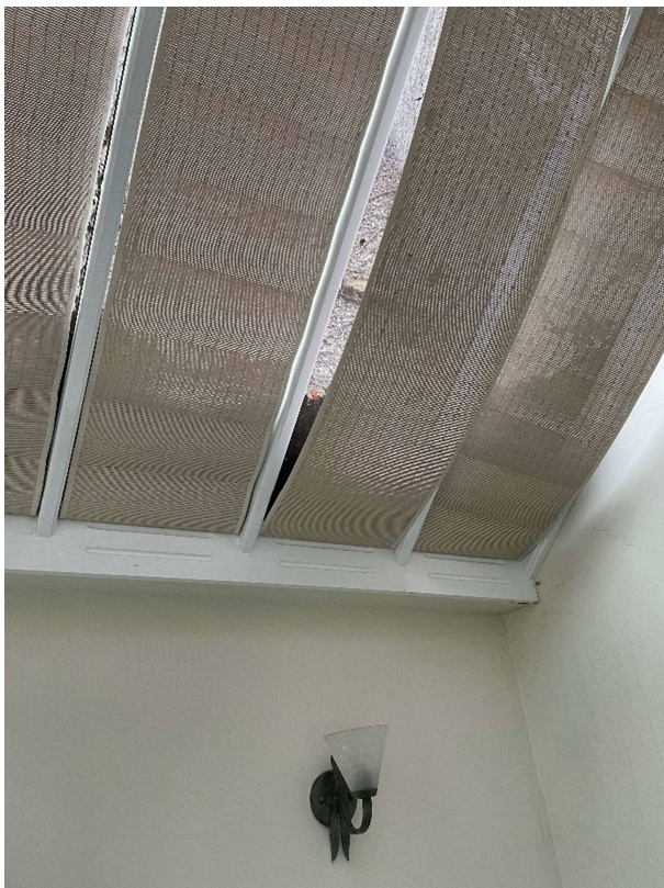
Photo 7. Internal photo showing build-up of leaves and debris in side gutter.
