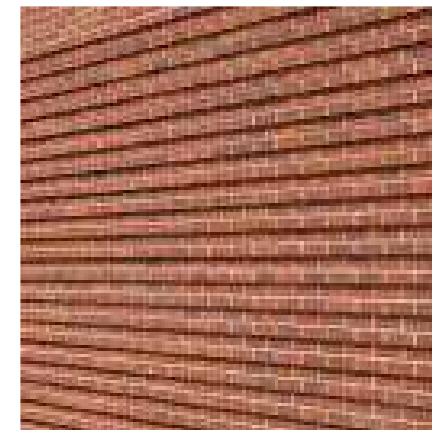
Red Brickwork Detailing
