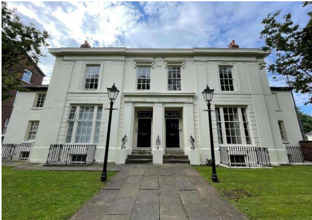
Figure 2.4: Principal Façade of 466-468 Moss Lane East
