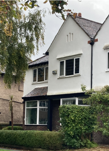
Example of Bellmouth detailing on Claude Road common to Chorltonville to be retained.
